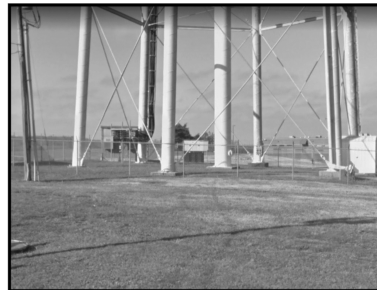
GROUND VIEW - DETENTION CENTER TANK
