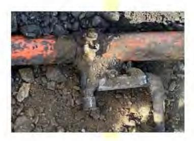
A leak like this on the Frontier system has 4 to 9x the effect on Frontier L&U as the same exact leak has on Atmos or LG&E or 2x as Burkesville or Delta
