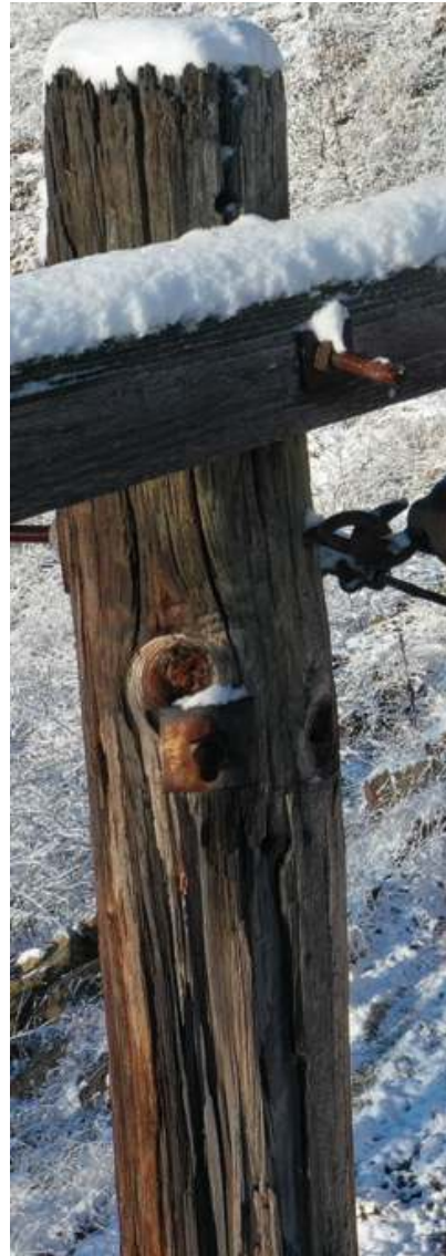
Structure K426-37: - Upper Pole Splitting
