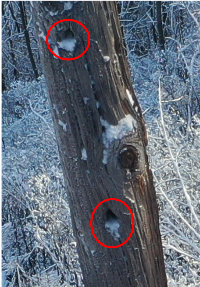
Structure K426-54: - Pole Cavities
