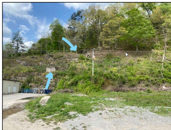
Photograph 2. Alternative Site A field review, facing west
