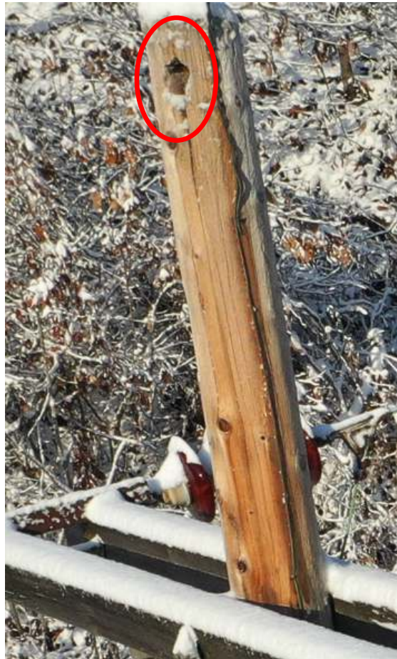
Structure K426-11: - Pole Cavity
