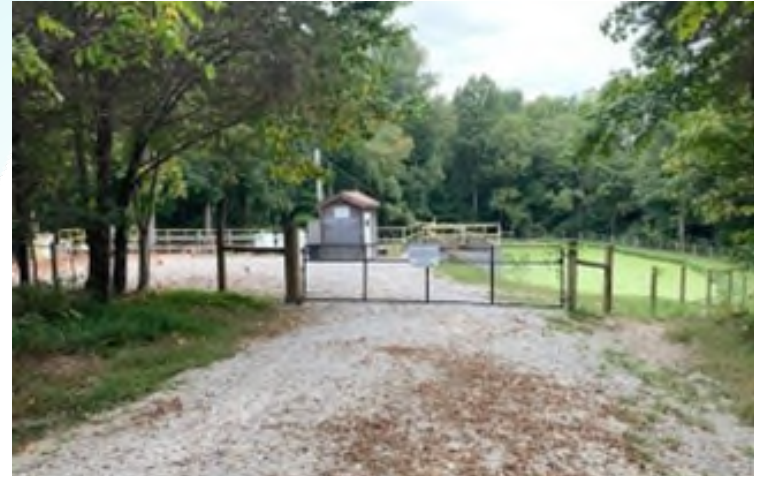
After: New fencing, recoated tank
