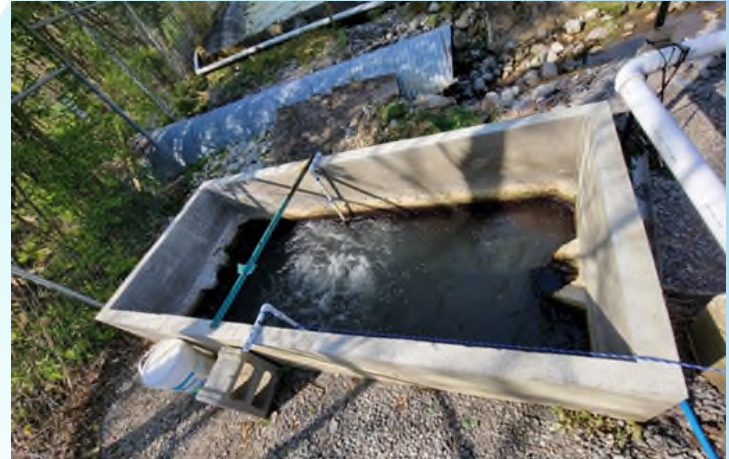
After: New contact chamber, erosion control implemented
