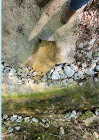
After: Improved effluent quality, new aeration piping
