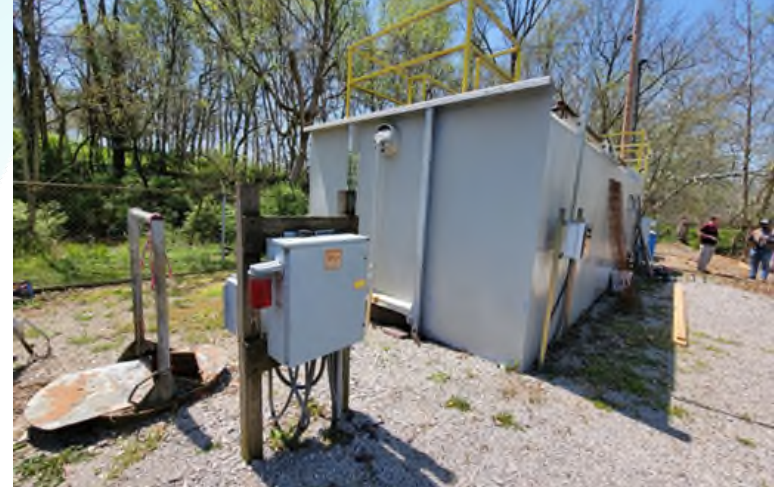
After: Improved influent lift station, safety rails installed
