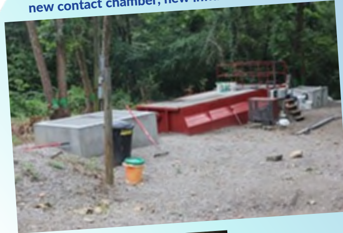
Before: Deteriorating aeration plant, deteriorated low functioning contact chamber & influence screen box
