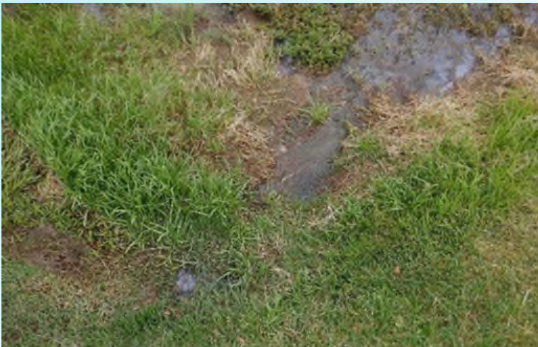
Before: Leaking, eroding, vegetation growing in berms
