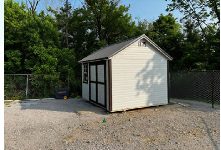
After: New disinfection shed, safety rails installed around treatment basin
