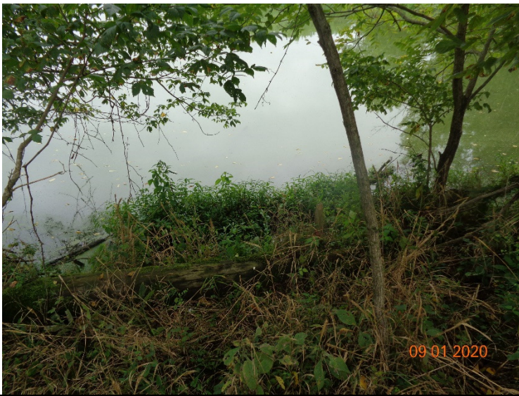
PRINCIPAL SPILLWAY PIPE OUTLET INTO LAKE BELOW
