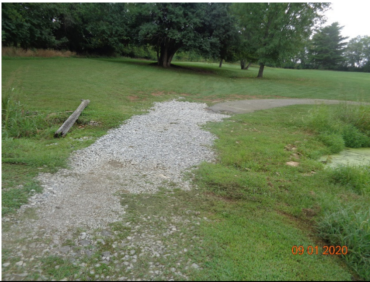
AUXILIARY SPILLWAY CONTROL SECTION
