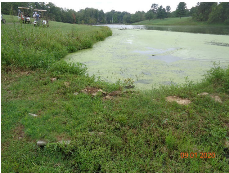
AUXILIARY SPILLWAY INLET
