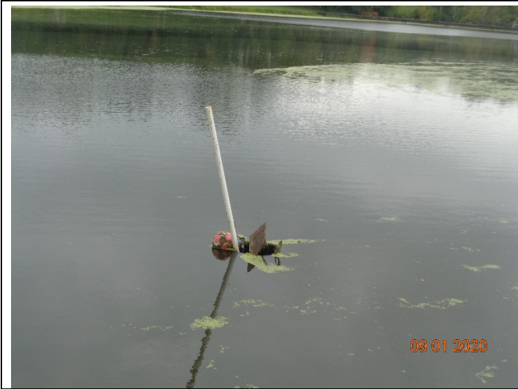
PRINCIPAL SPILLWAY HOODED INLET
