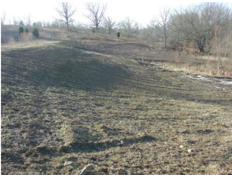
2009 PHOTO - DOWNSTREAM SLOPE IS CLEARED OF ALL BRUSH AND TREES
