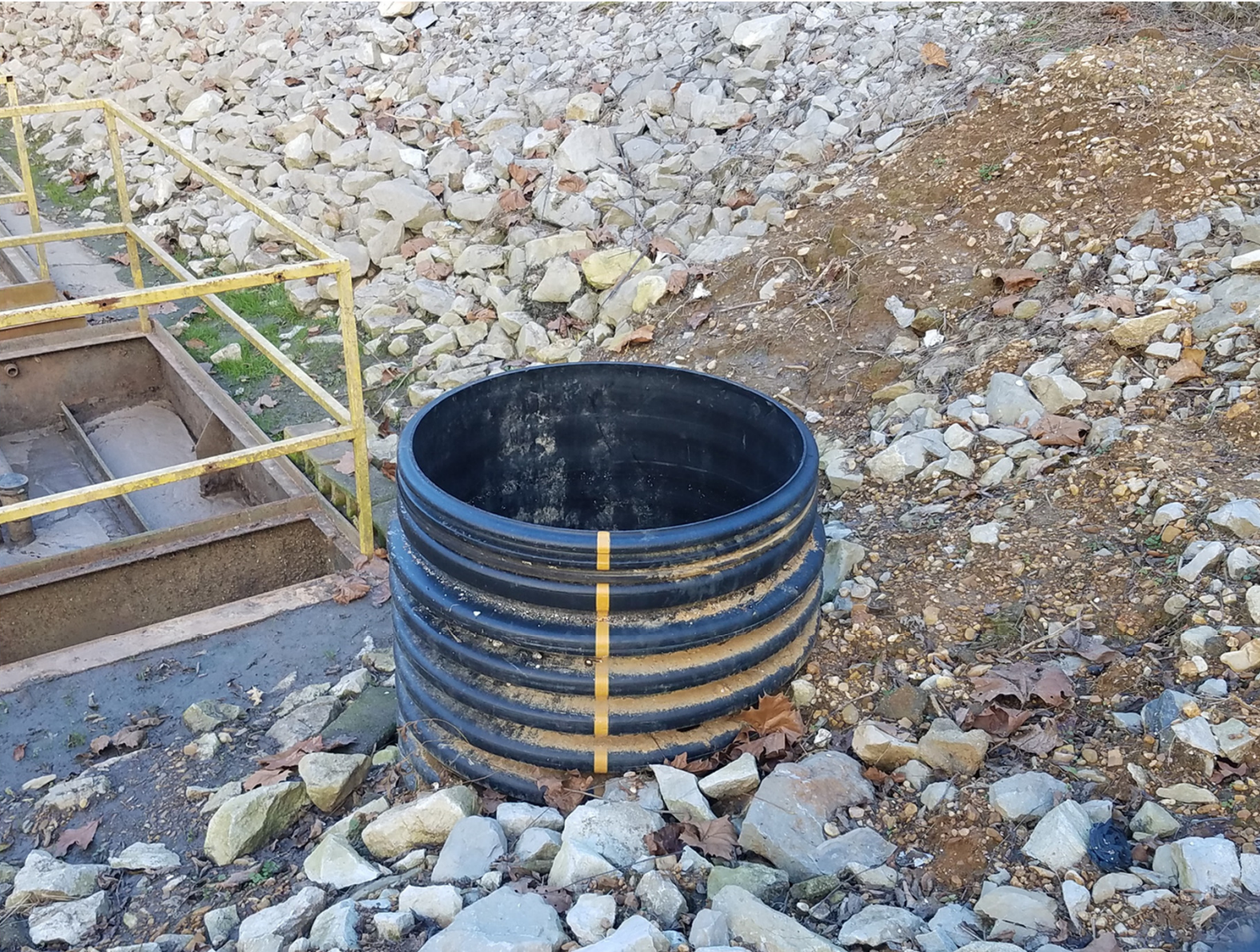
Flow meter housing
