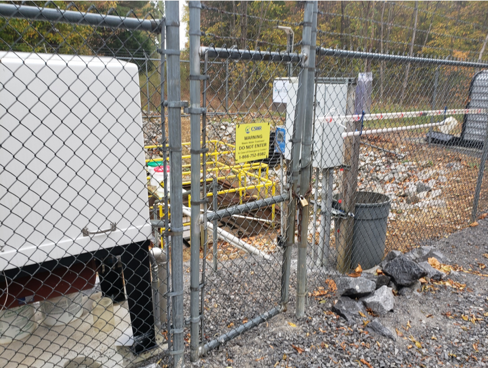
Secure fence with locked gate
