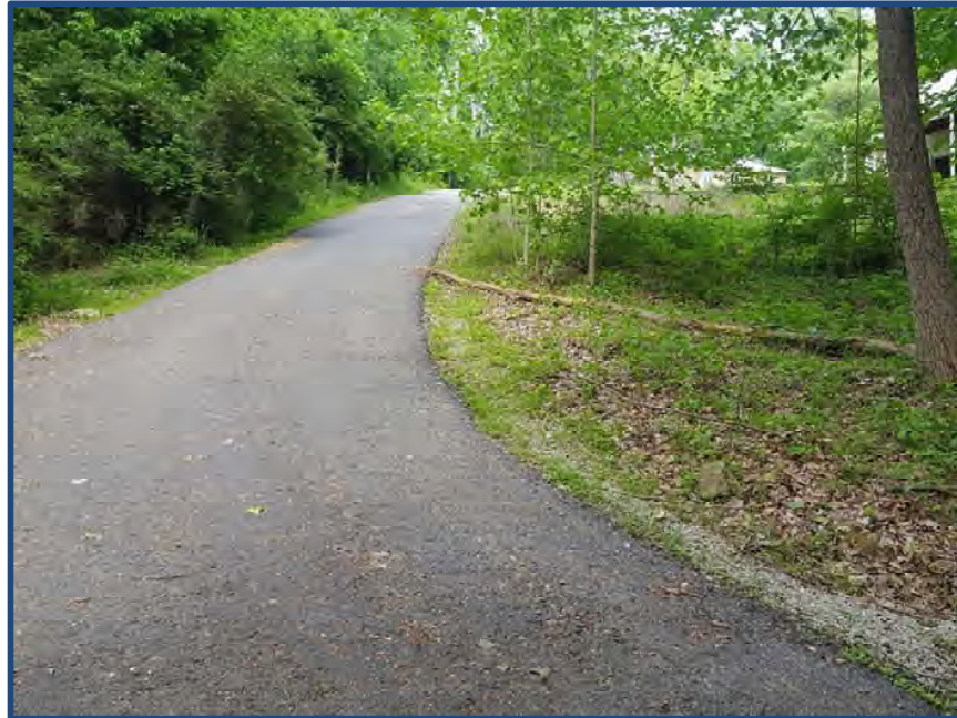
View looking along access drive toward Creekview Road
