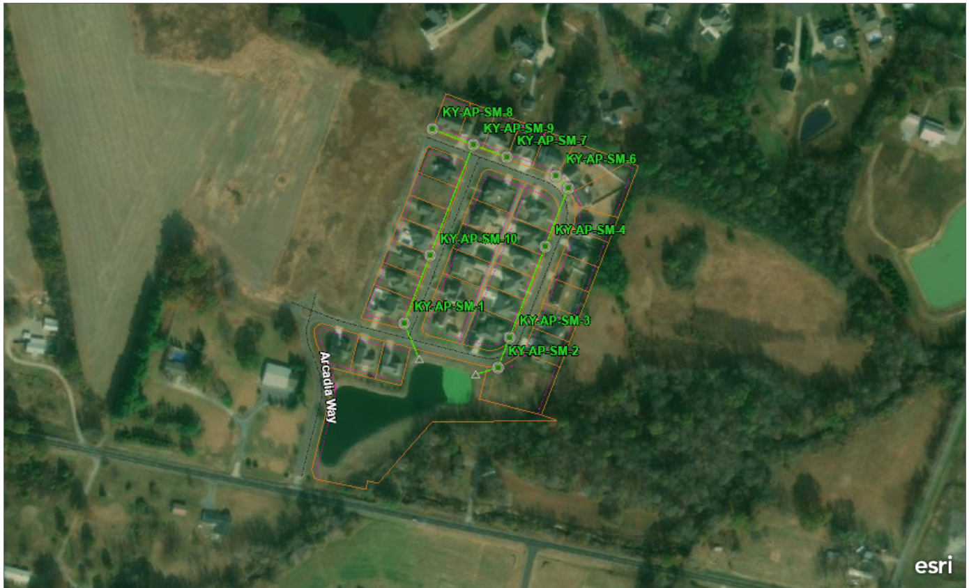
Arcadia Pines Subdivision wastewater system in McCracken County, Kentucky.
