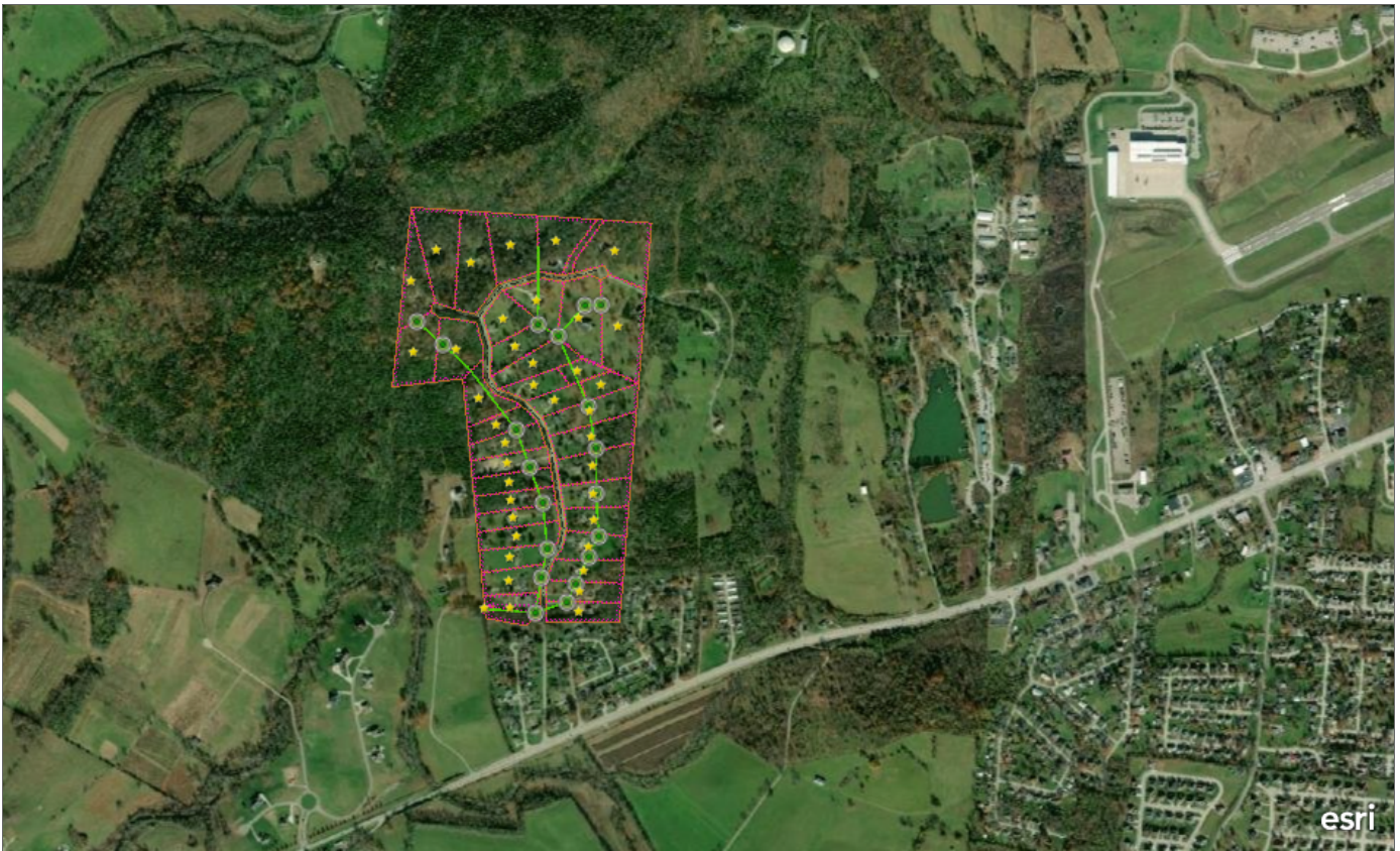
Fox Run Estates wastewater system in Franklin County, Kentucky
