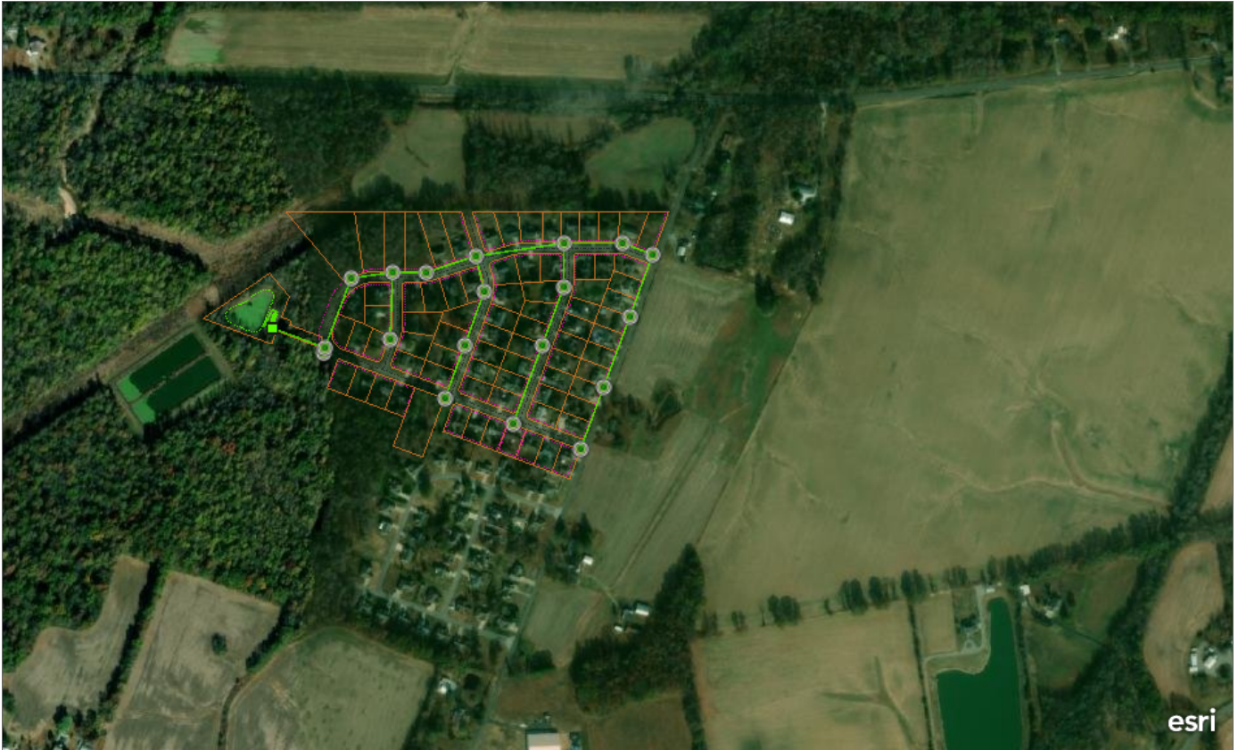
Timberland Subdivision wastewater system in McCracken County, Kentucky.
