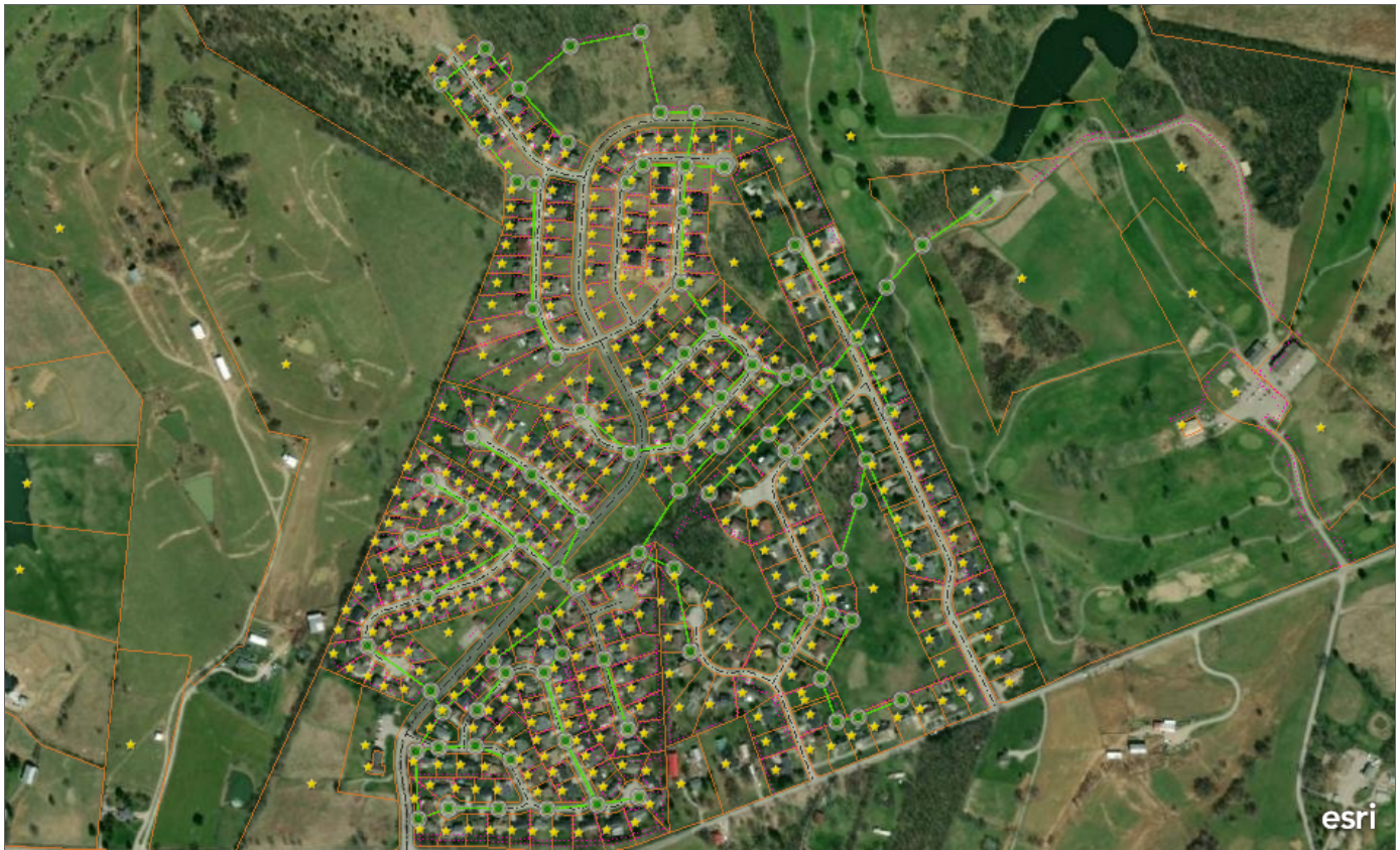
The Homestead and Longview Estates wastewater system in Scott County, Kentucky
