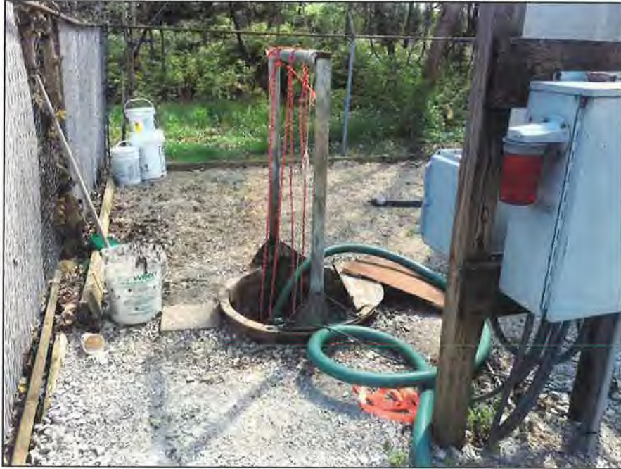
Lift station with a sump pump. Lift station needs a cover. Electrical cord needs to be properly protected from the elements.
