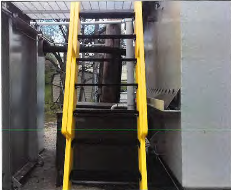
New stairs leading to the top of the plant
