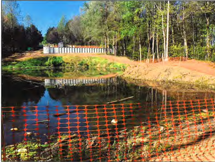
Airview Wastewater Treatment Facility
