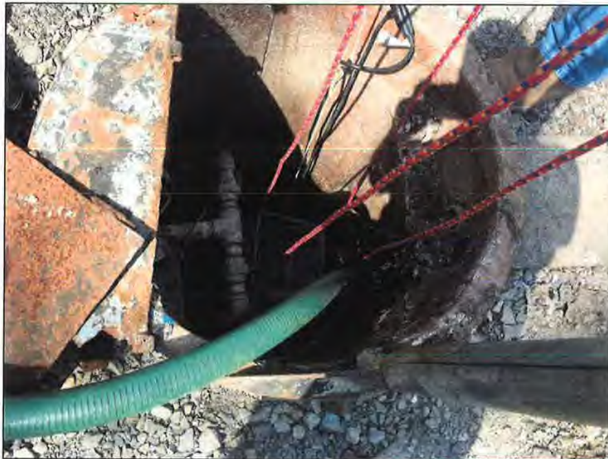
Lift station with a sump pump. Lift station needs a cover. Electrical cord needs to be properly protected from the elements.
