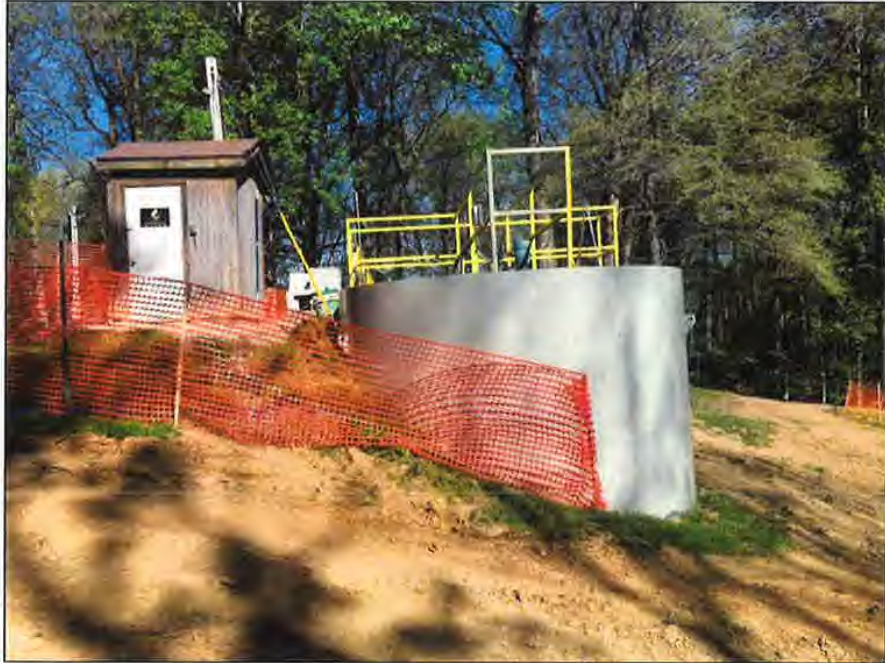
Outside walls of Clarifier newly painted
