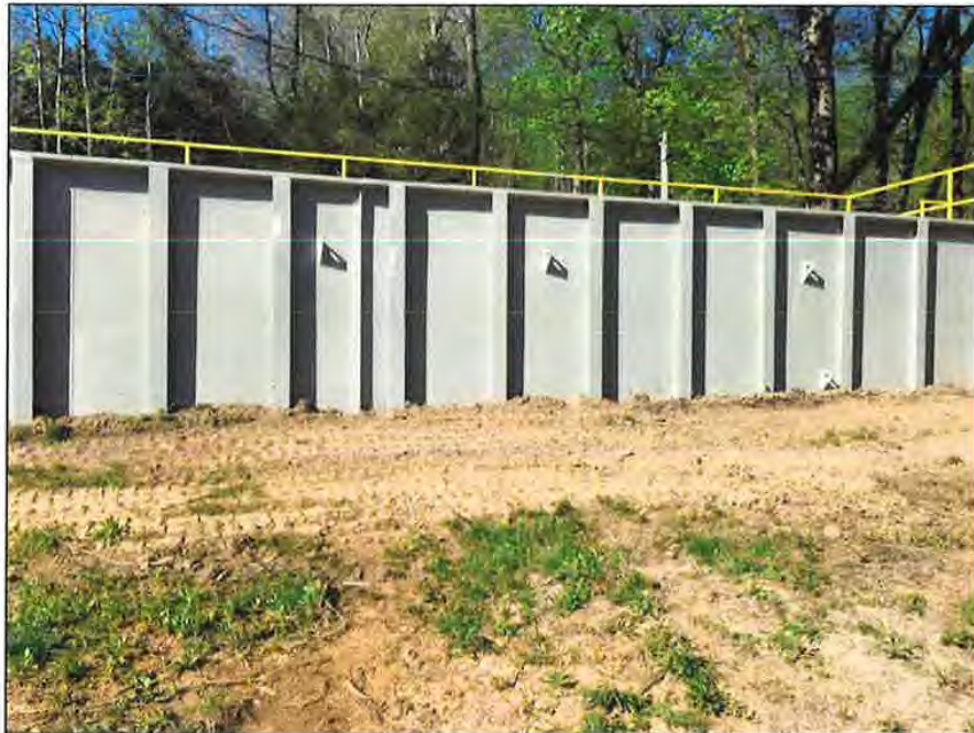
Outside walls of treatment Plant newly painted
