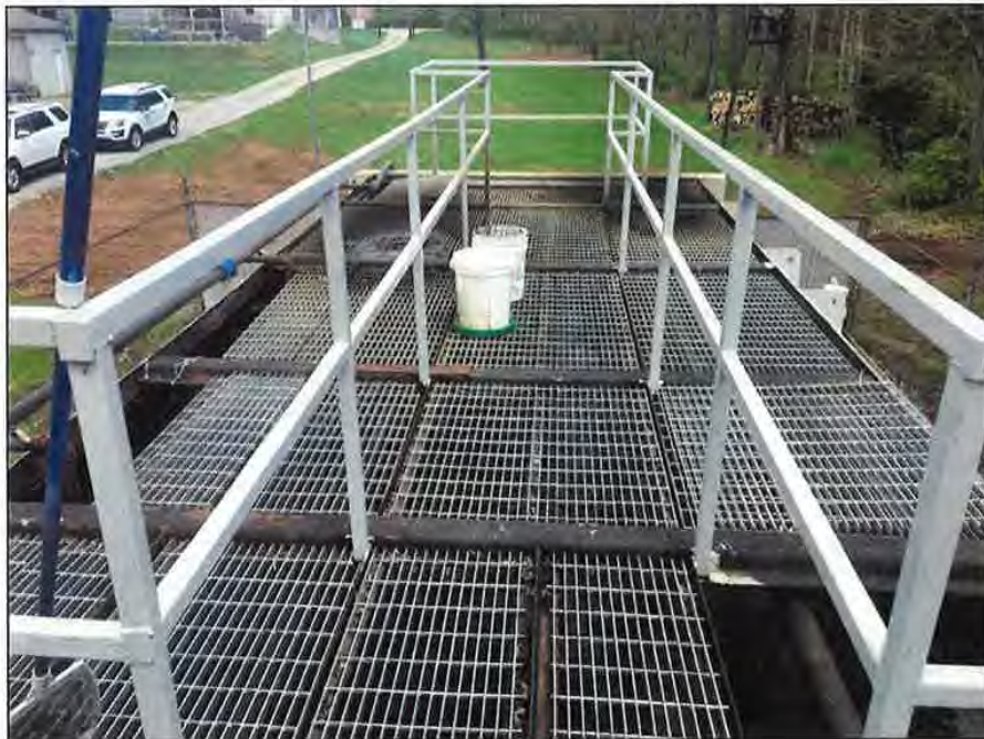
Safety Rails Added to the Plant
