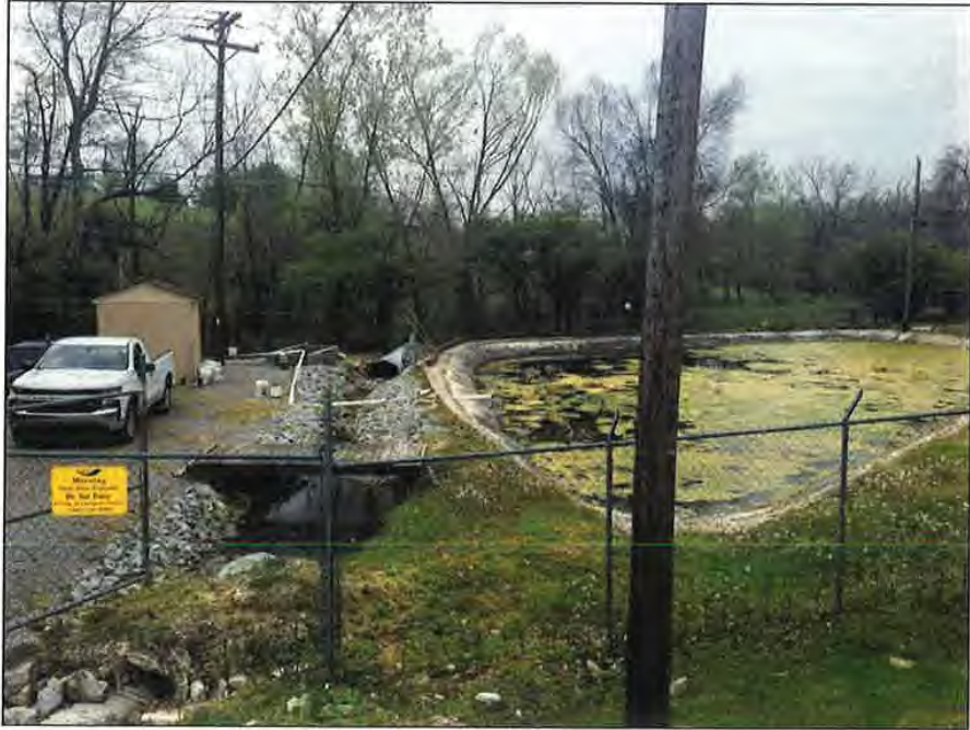
Storm water drainage
