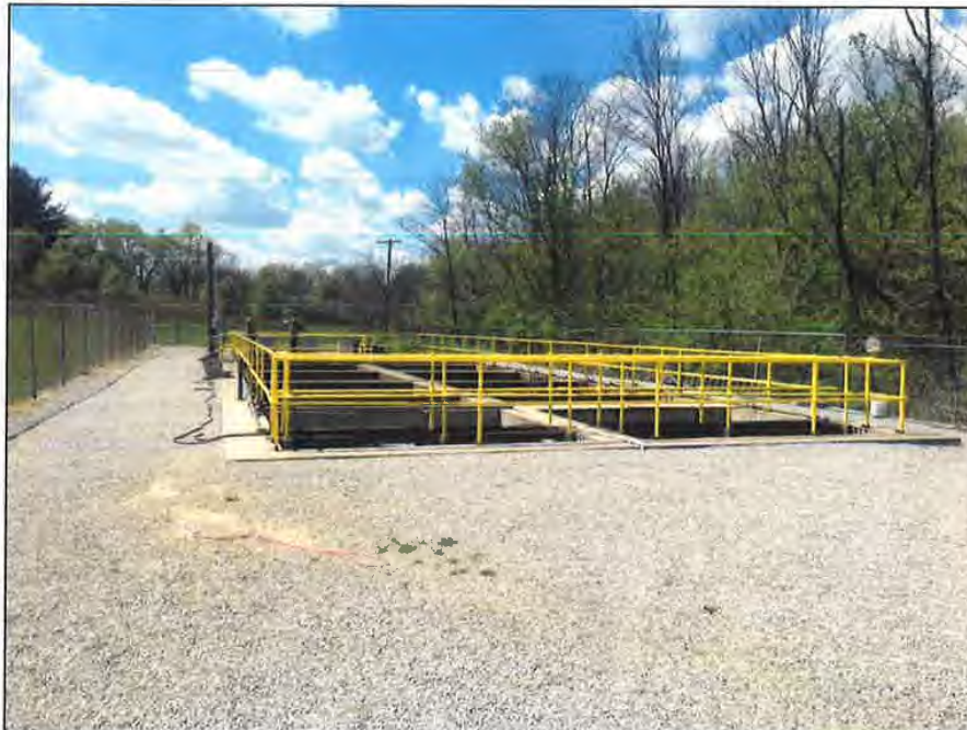
Safety Rails have been added
