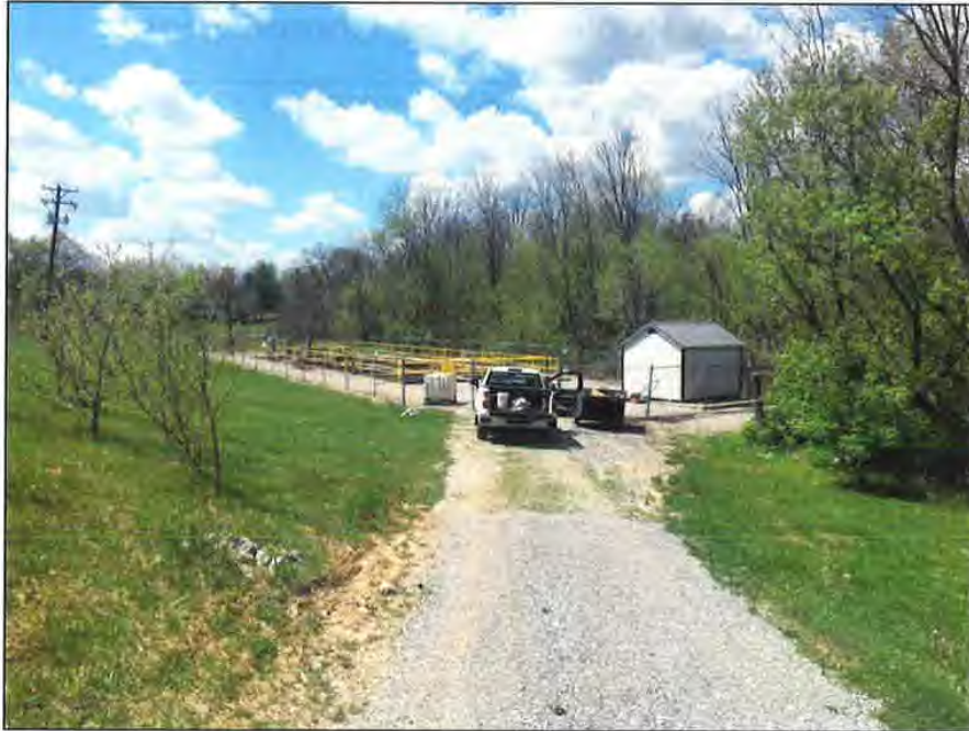
Longview Wastewater Treatment Plant
