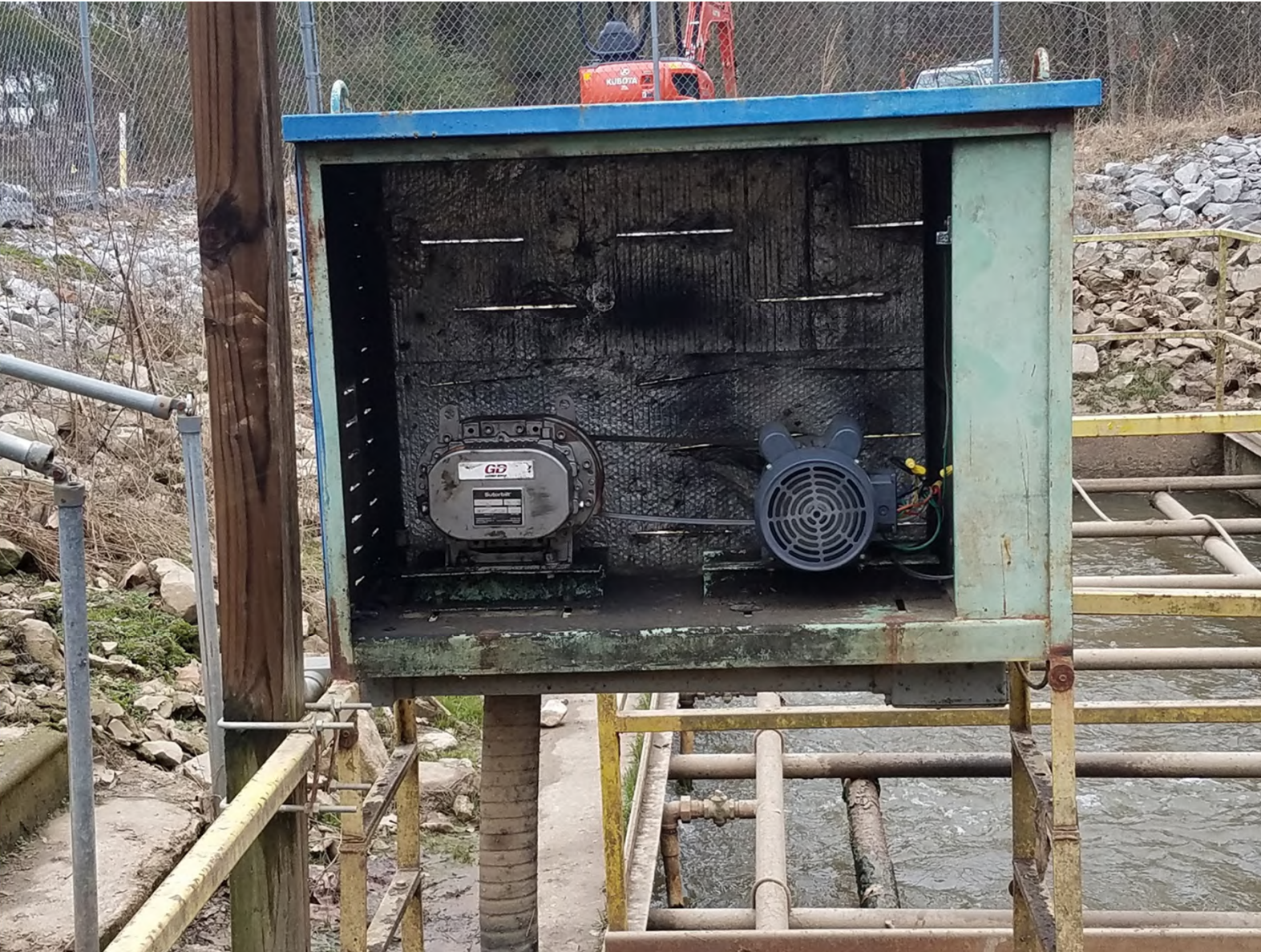
New motor for aeration pump.
