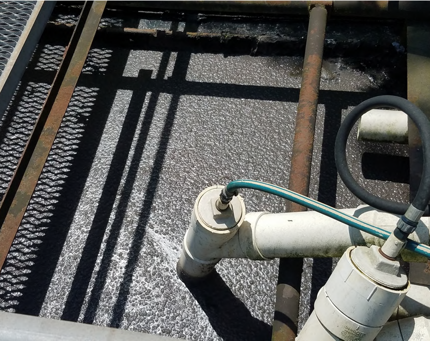
Excessive nitrification in the clarifier
