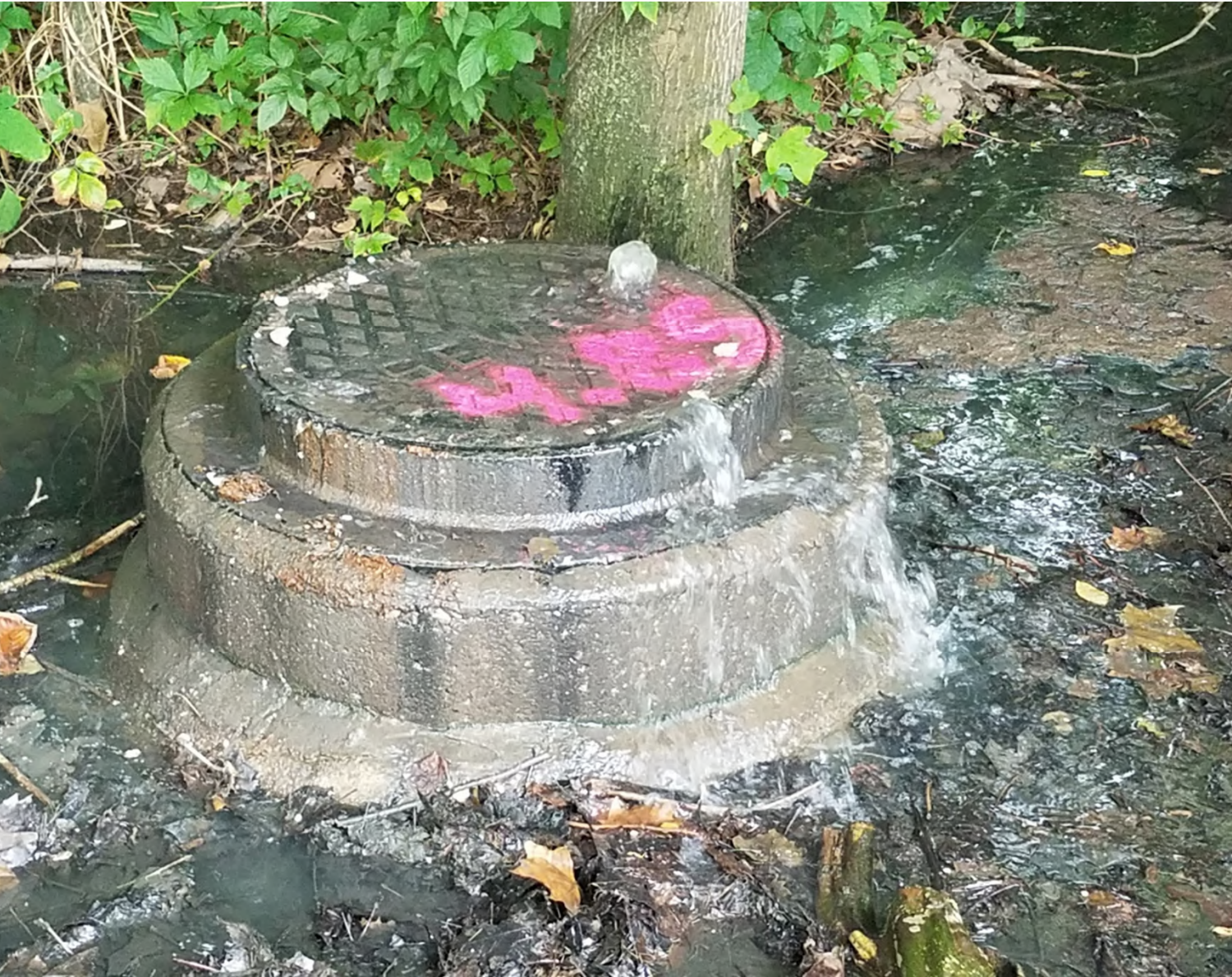
Manhole at 5730 Majestic Oak Drive
