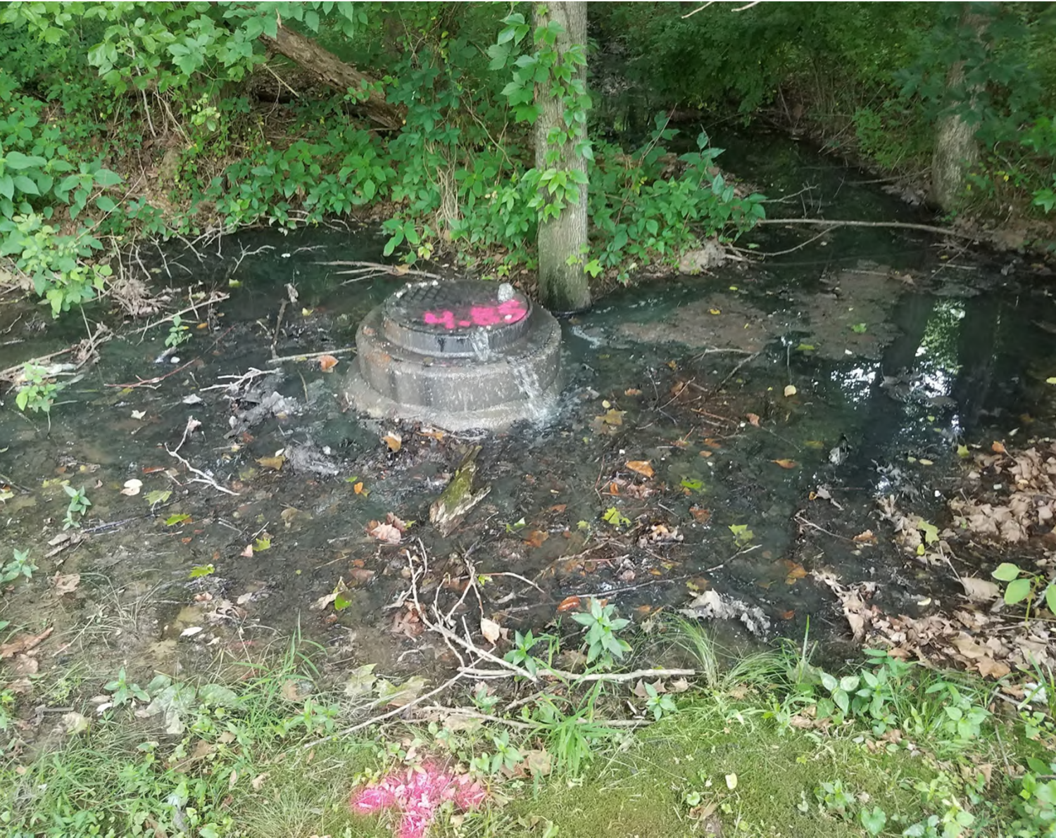
Manhole at 5730 Majestic Oak Drive
