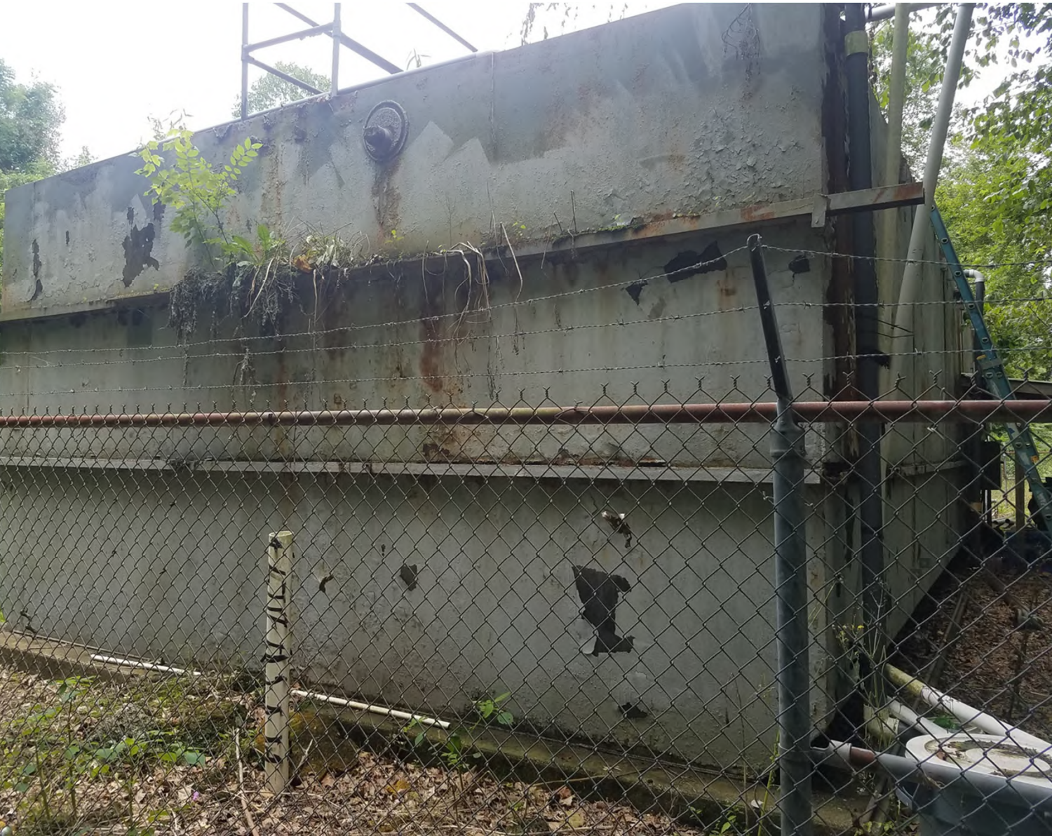
Solids on the side of the plant
