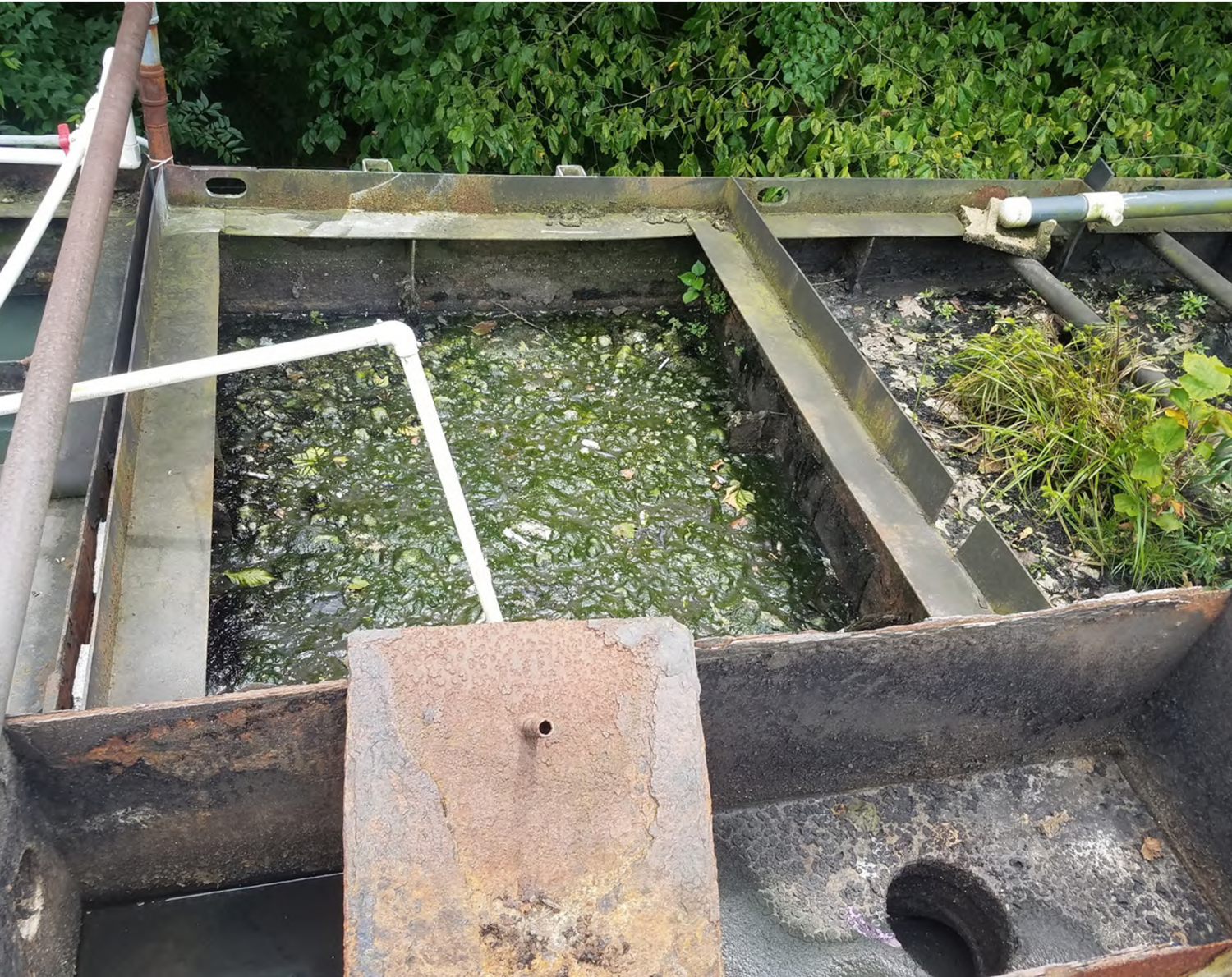
Solids in the aeration basin
