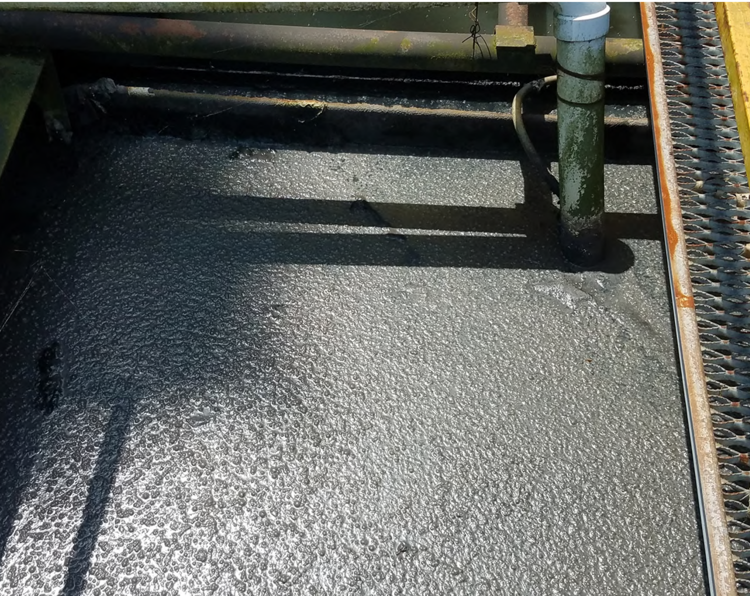
Excessive nitrification in the clarifier
