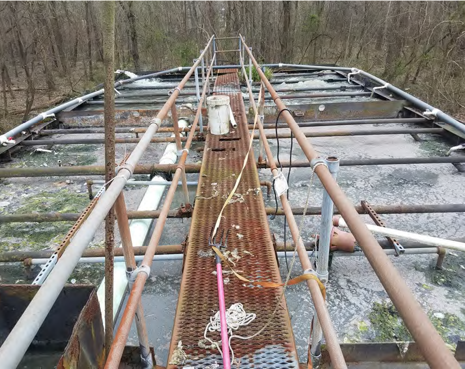
Solid cap over large portion of the aerator
