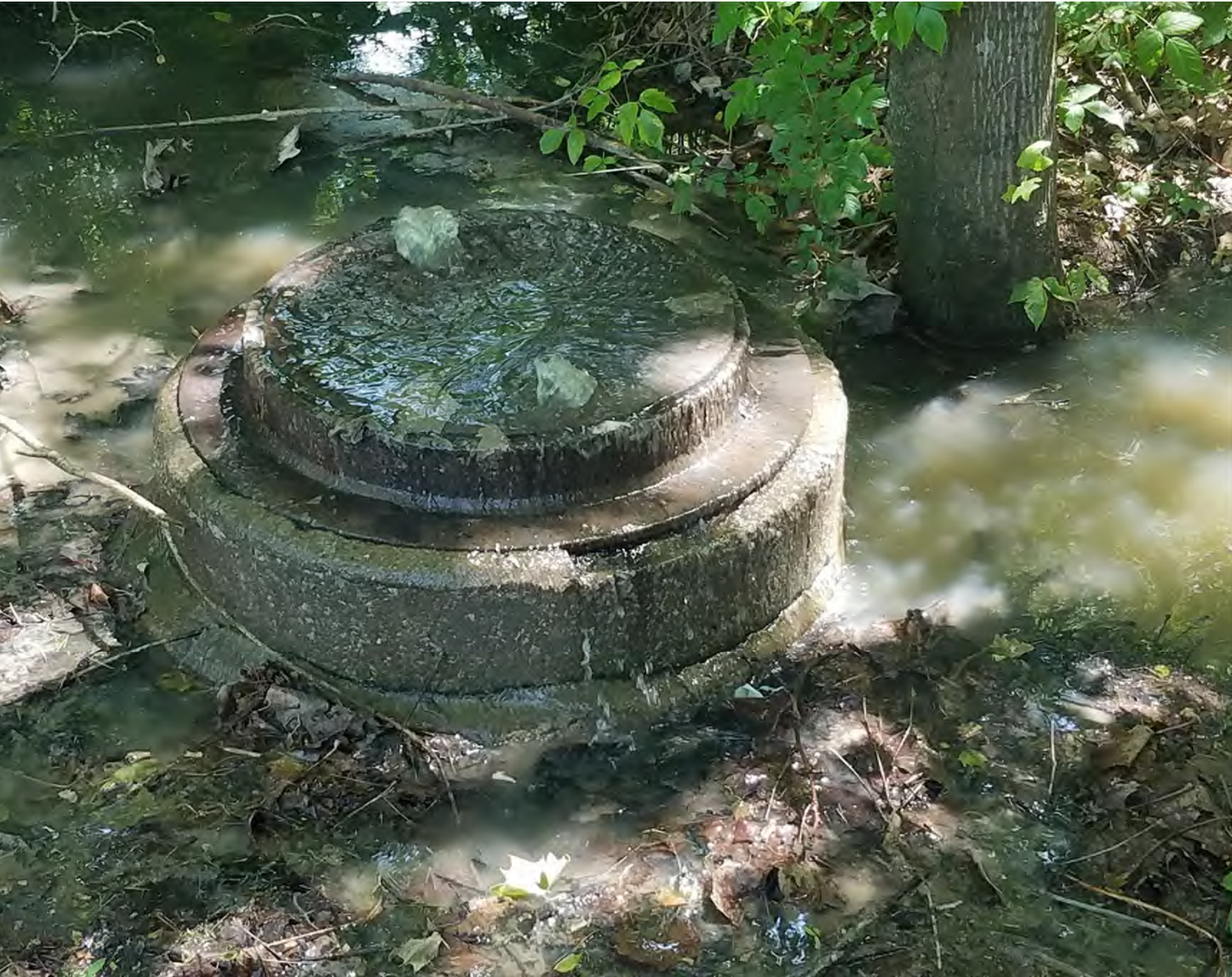
Manhole at 5730 Majestic Oak Drive
