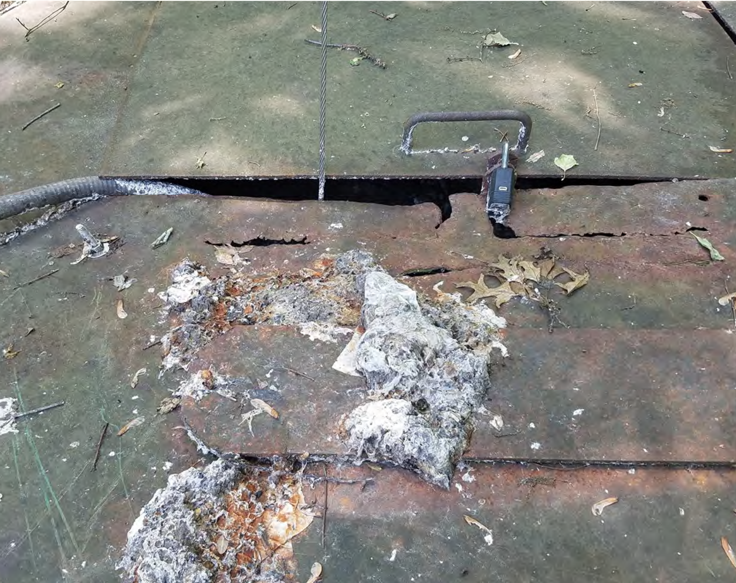
Solids on the lift station
