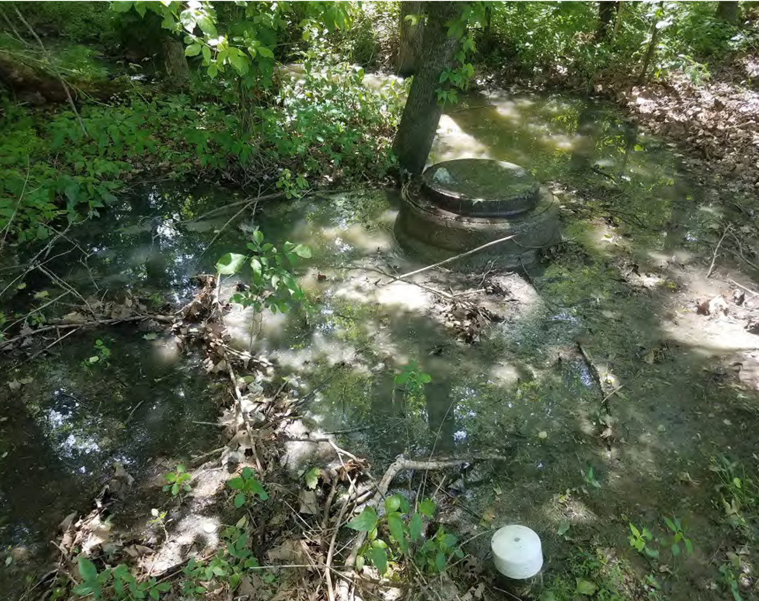
Manhole at 5730 Majestic Oak Drive
