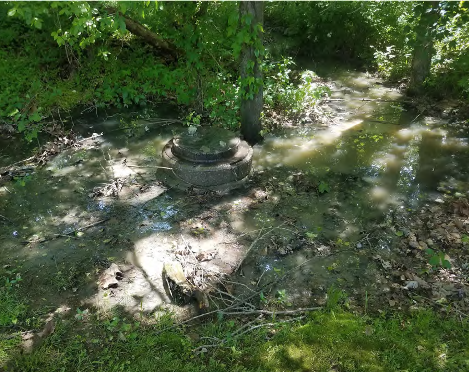
Manhole at 5730 Majestic Oak Drive
