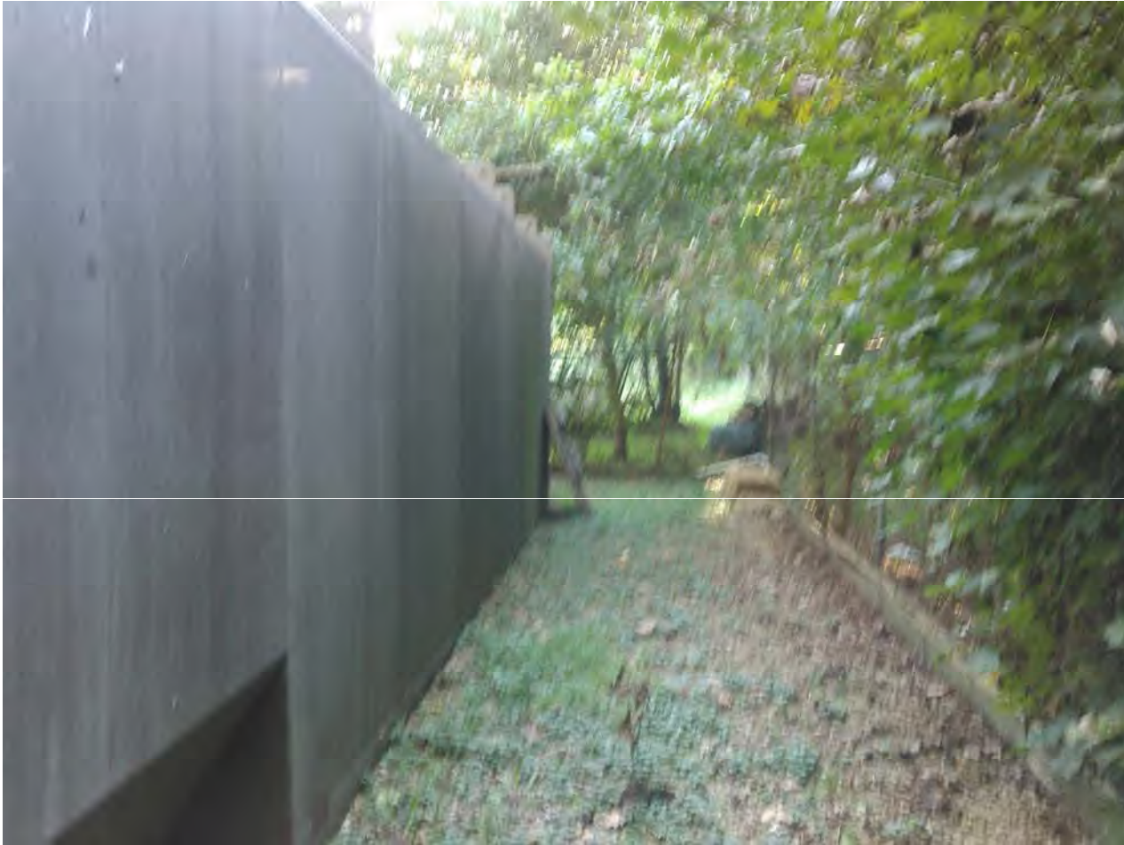
Fox Run WWTP, Frankfort, KY September 17, 2015. Deborah Singleton, Environmental Inspector. View of plant.
