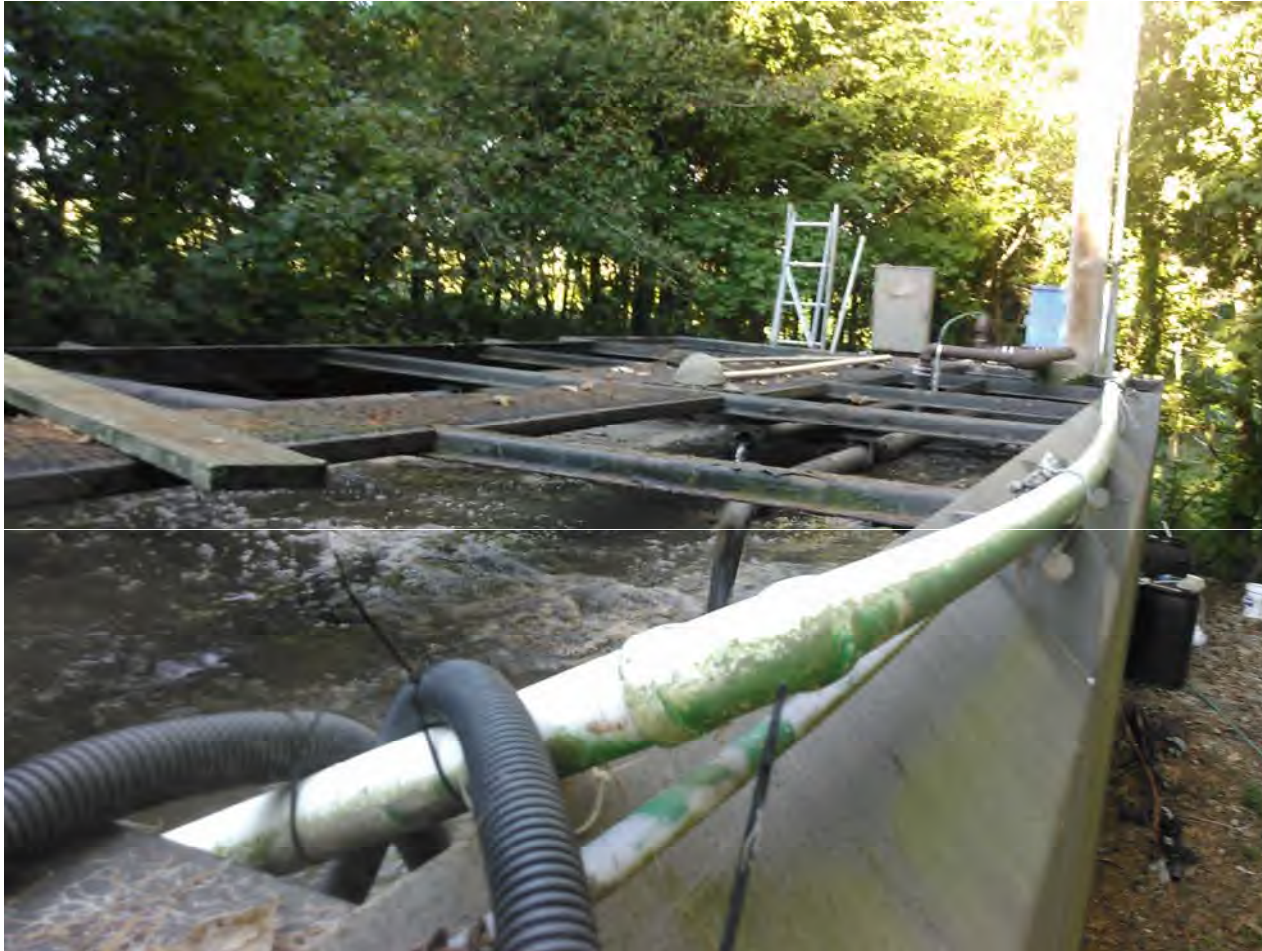
Fox Run WWTP, Frankfort, KY September 17, 2015. Deborah Singleton, Environmental Inspector. Aeration basin had good roll and color.
