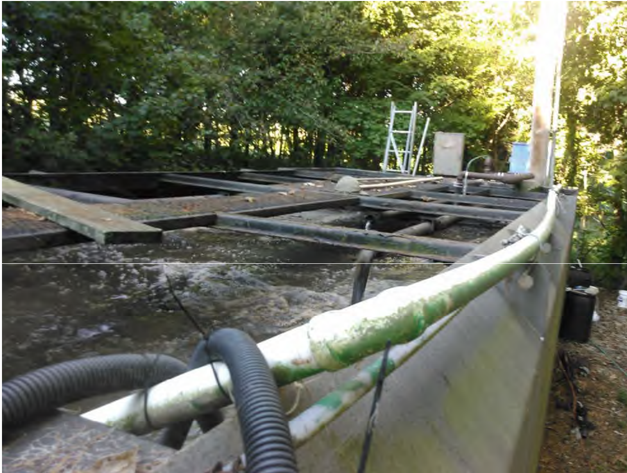
Fox Run WWTP, Frankfort, KY September 17, 2015. Deborah Singleton, Environmental Inspector. Aeration basin had good roll and color.
