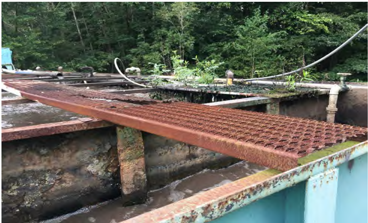
Bar Screen with vegetation and sludge. Grating appears unsafe to walk on.
