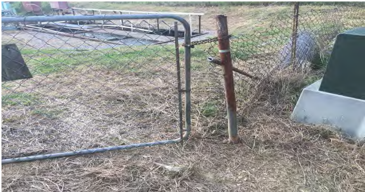
Gap between the fence post and gate
