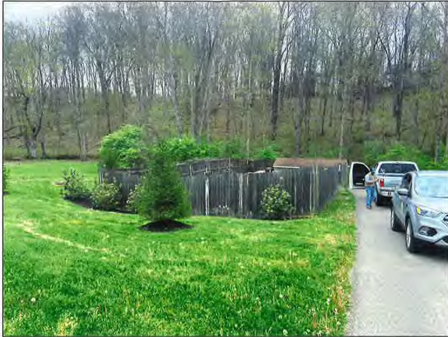
Darlington Creek HOA WWTP
