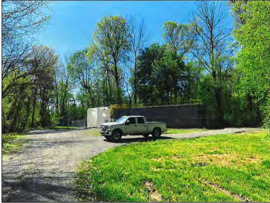
Great Oaks WWTP
