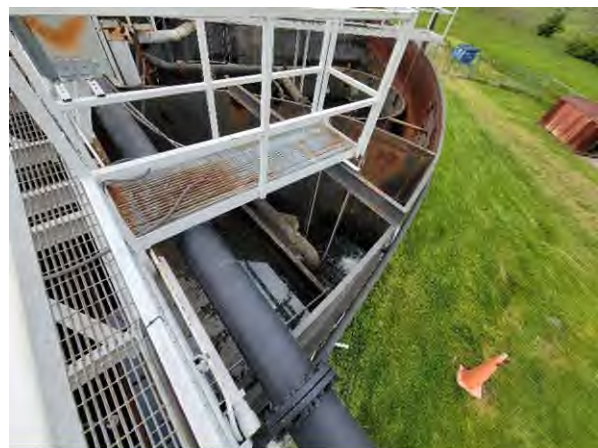
Notable rust on air header, walkways, tank, and transfer piping.
