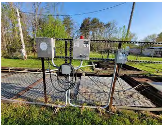
15 New handrails and basin covers installed for operator safety.
