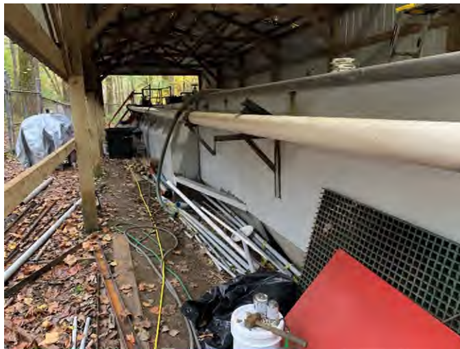
Repaired tank exterior.
