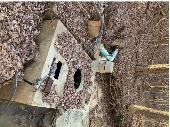
Before and after contact chamber removal and new dechlorination tablet feeder
