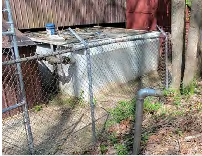
Repaired and recoated sludge holding tank.
