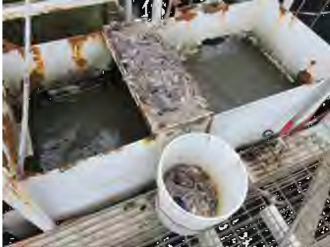
Examples of nuisance solids at Delaplain.
