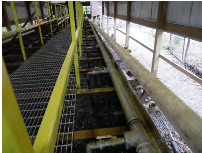
12 New aeration piping (header drops and valving), new catwalk and handrails. 13 14
