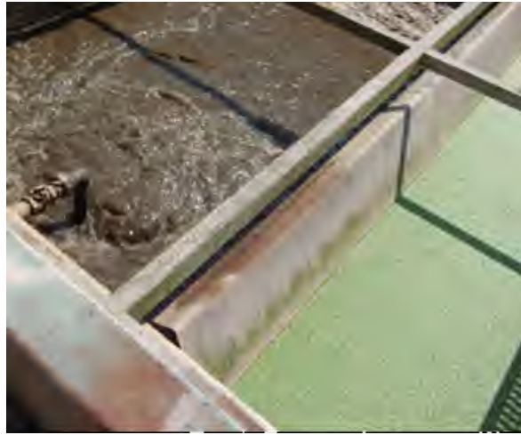
3 4 Thick layer of duckweed in clarifier indicating scum return failure.
