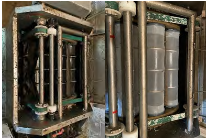
9 10 Darlington Creek tertiary filter before and after repairs.
