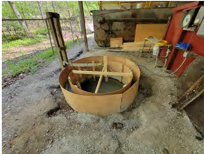
12 13 Form work for new dechlorination chamber.
