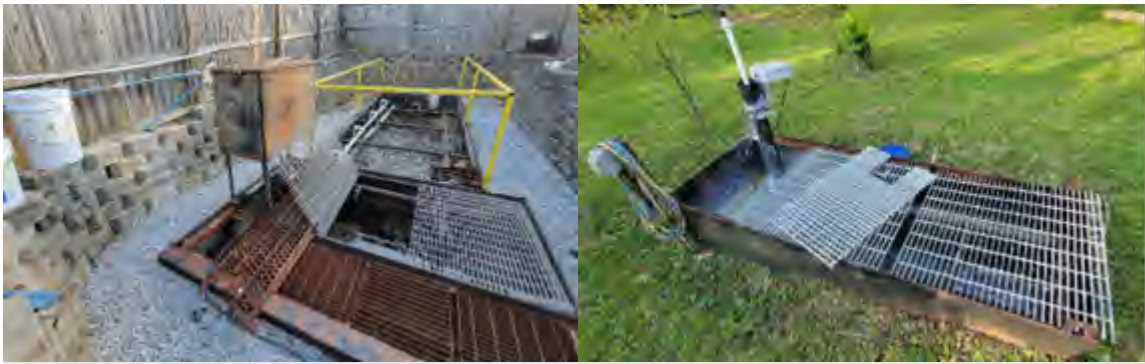
New handrails and basin cover installed for operator safety.
