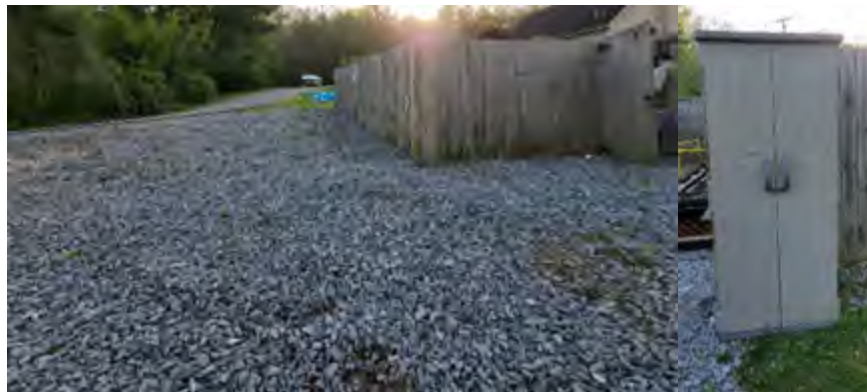
11 12 New rock applied to site and storage cabinet installed.
