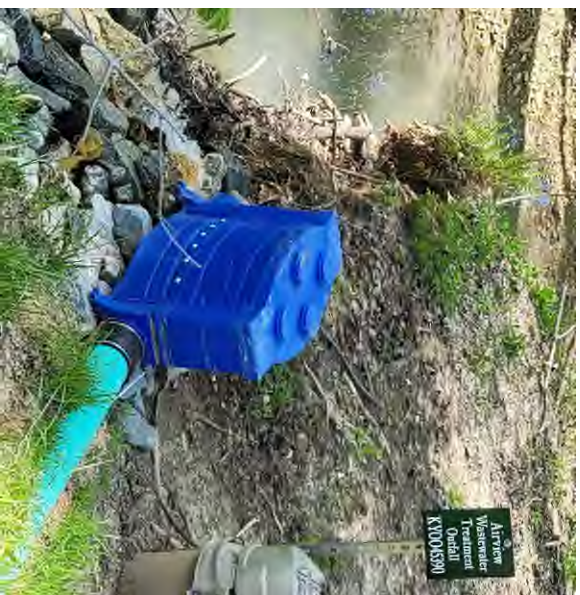
Before and after contact chamber removal and new dechlorination tablet feeder
