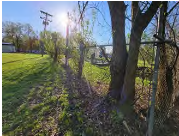
7 8 Trees and vegetation causing damage to facility fencing.
