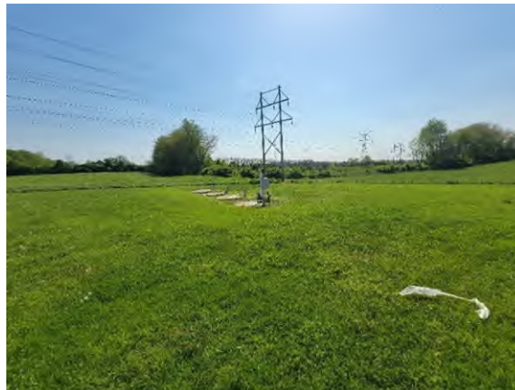
14 15 Drain field and wet well area mowed and being maintained.
