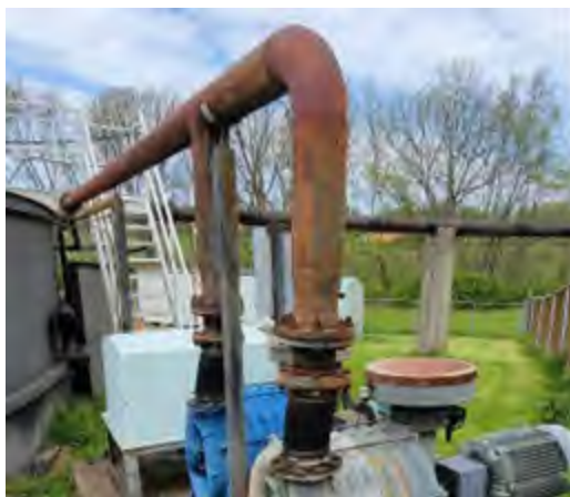
Notable rust on air header, walkways, tank, and transfer piping.
