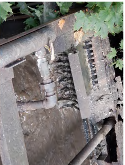
Before and after bar screen replacement.
