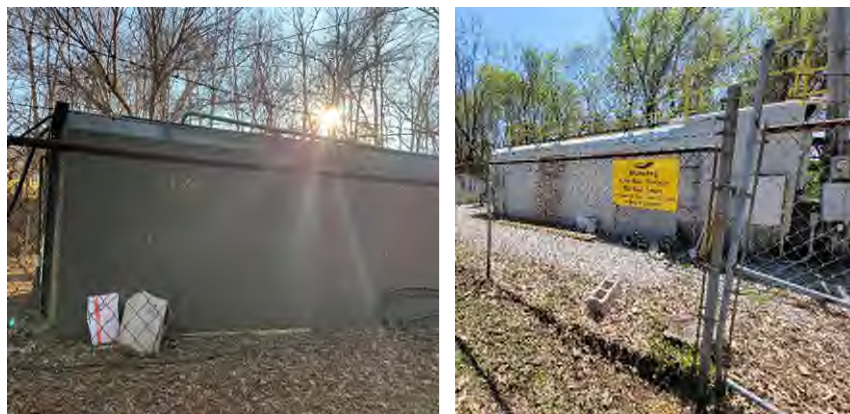
17 Before and after exterior repairs and coating, and handrail installation. 18
