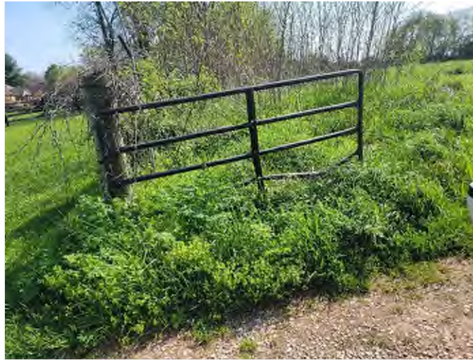
6 7 Condition of facility gate at acquisition.
