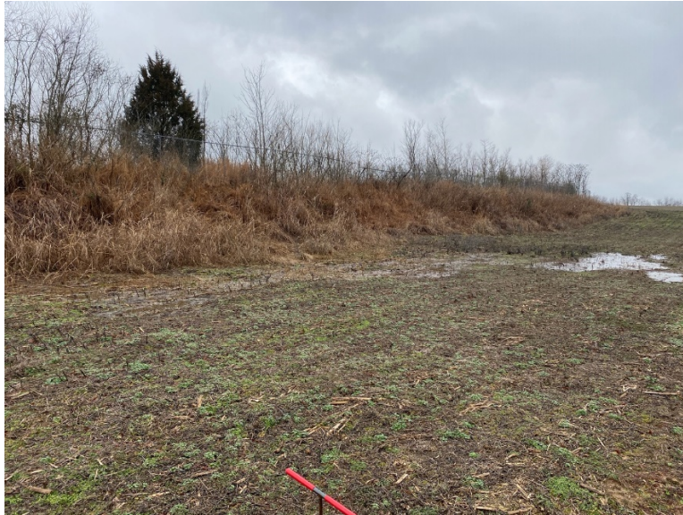
Lagoon seepage and overflow into crop field
