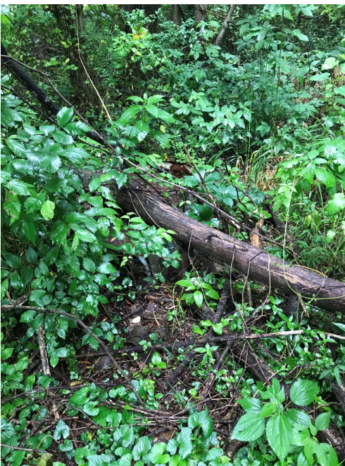
Tree fallen on lift station 1
