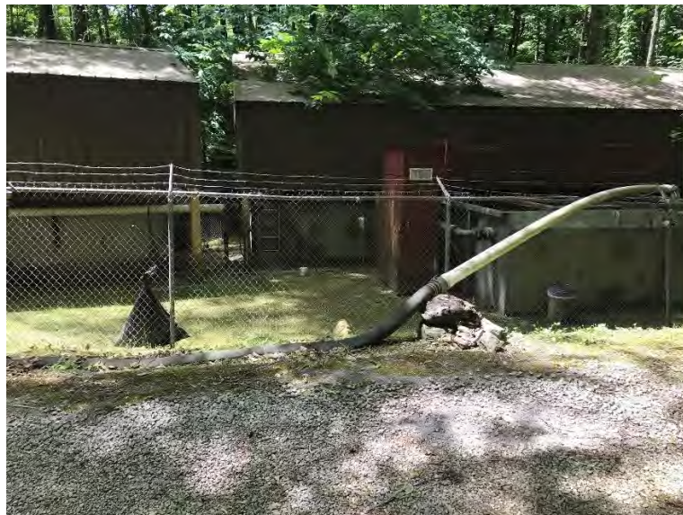
Influent PVC line is fastened to the top of the fence and should be properly buried.
