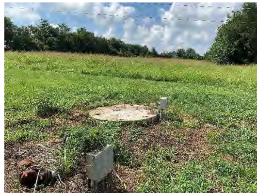
Triplex Irrigation Pump Station Nos. 3 & 4
