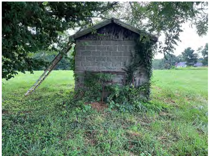
Electrical / Control Building and Irrigation Area in Background
