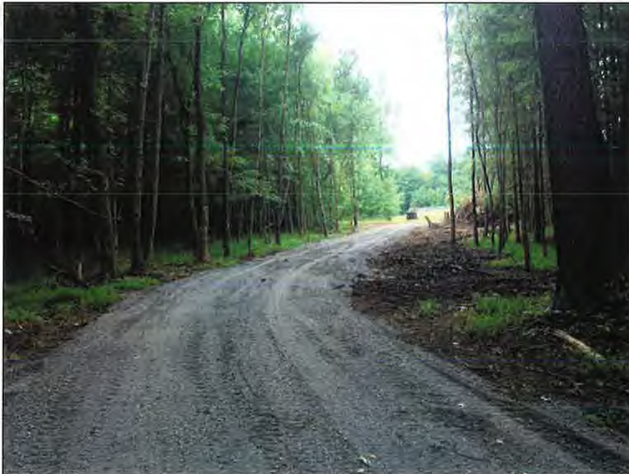
Construction of Access Road between Carriage Park WWTF and Timberland WWTF
