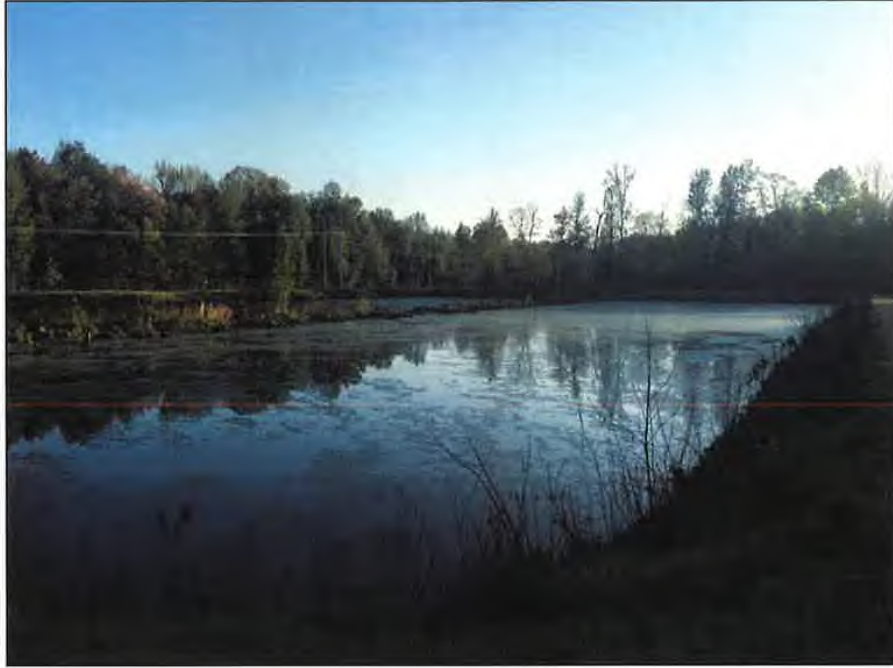
Carriage Park WWTF
