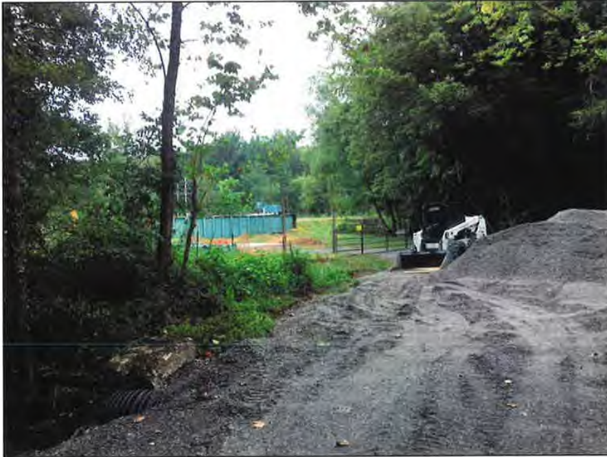
Access Road between Timberland and Carriage Park WWTF
