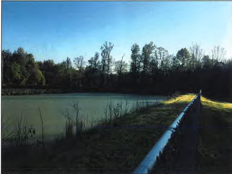
Carriage Park WWTF
