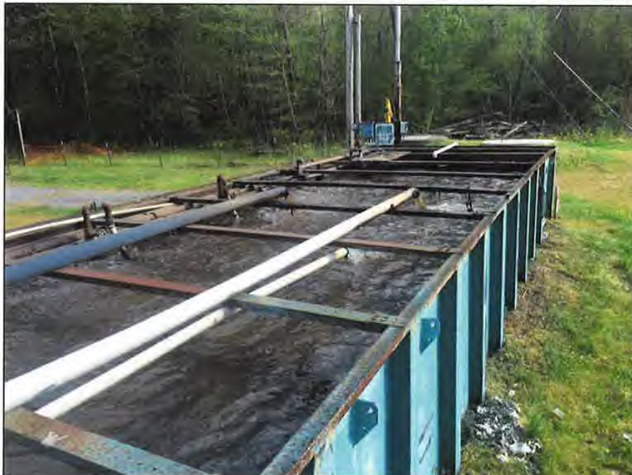
Wastewater Treatment Plant – Aeration Basin
