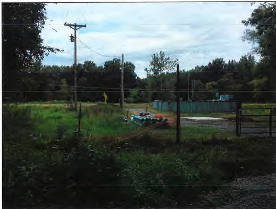
Timberland Wastewater Treatment Plant
