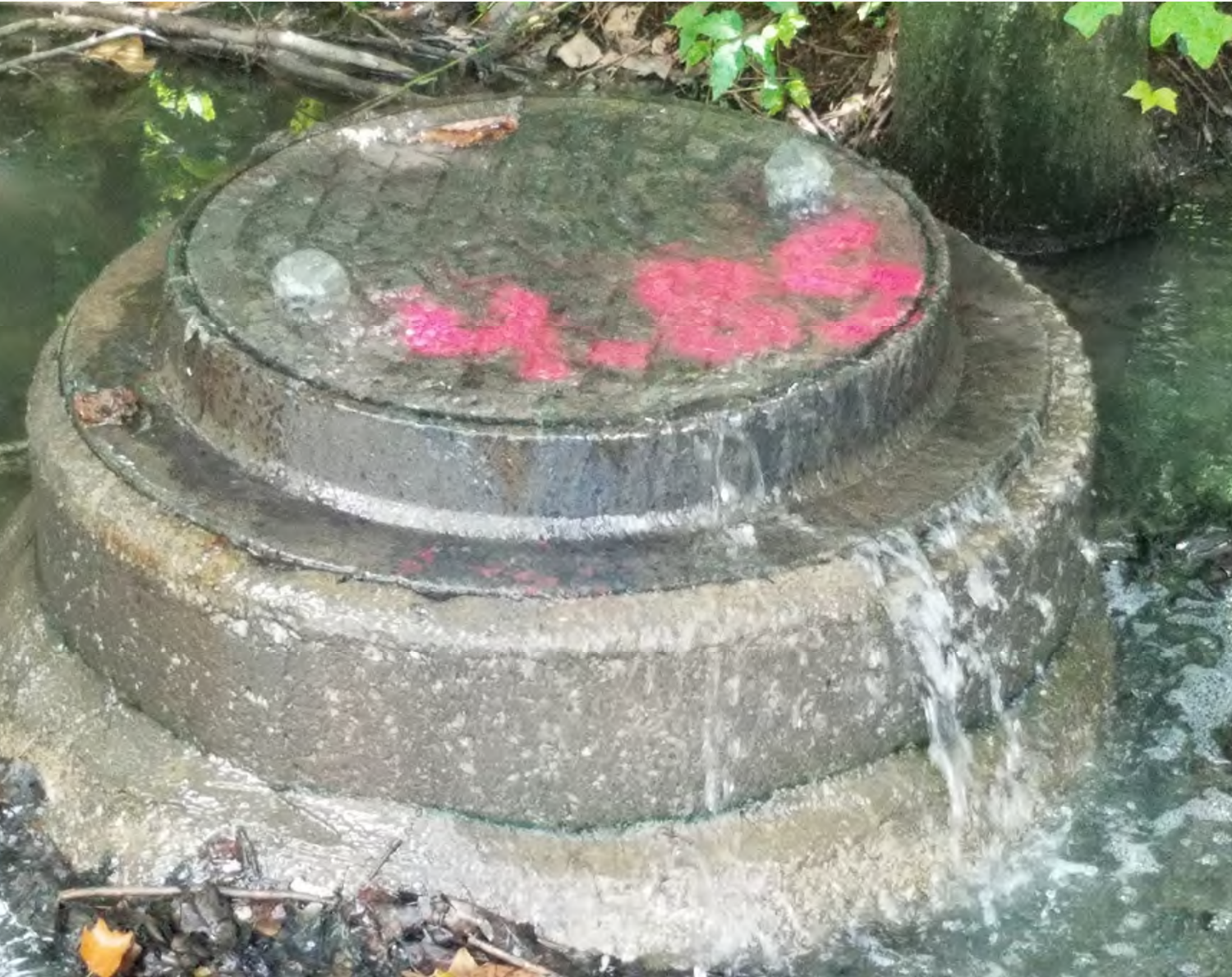
Manhole at 5730 Majestic Oak Drive
