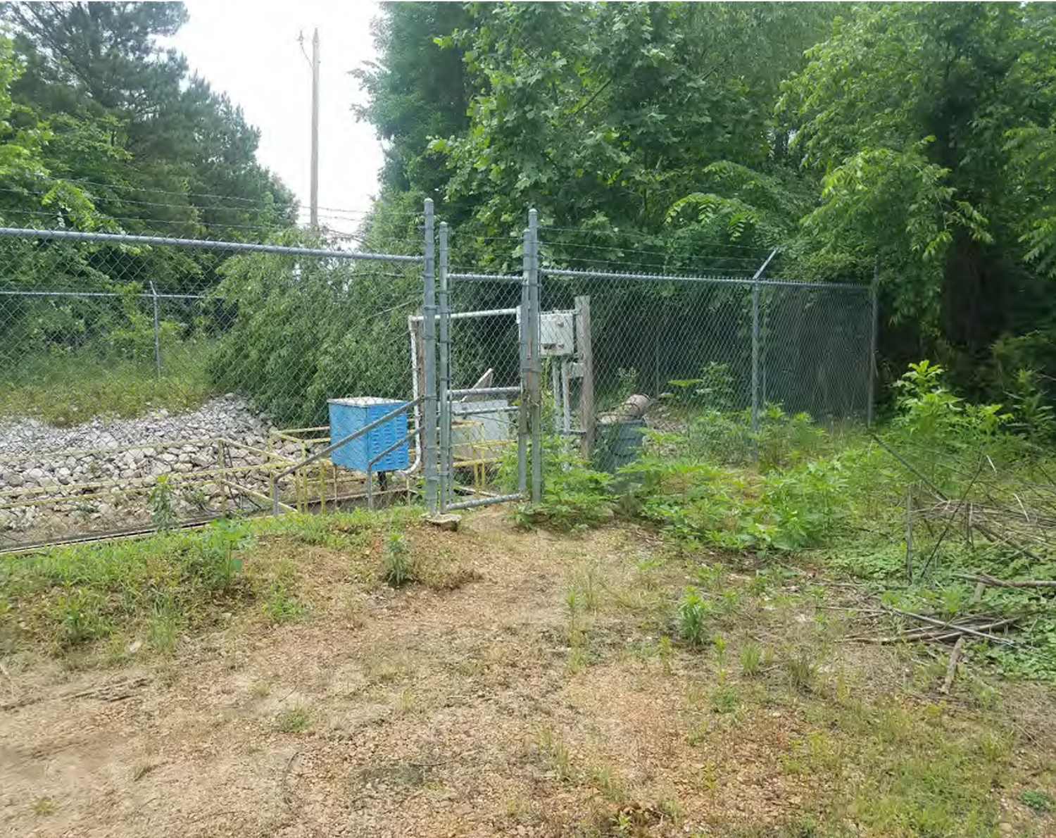
Fence with locked gate.
