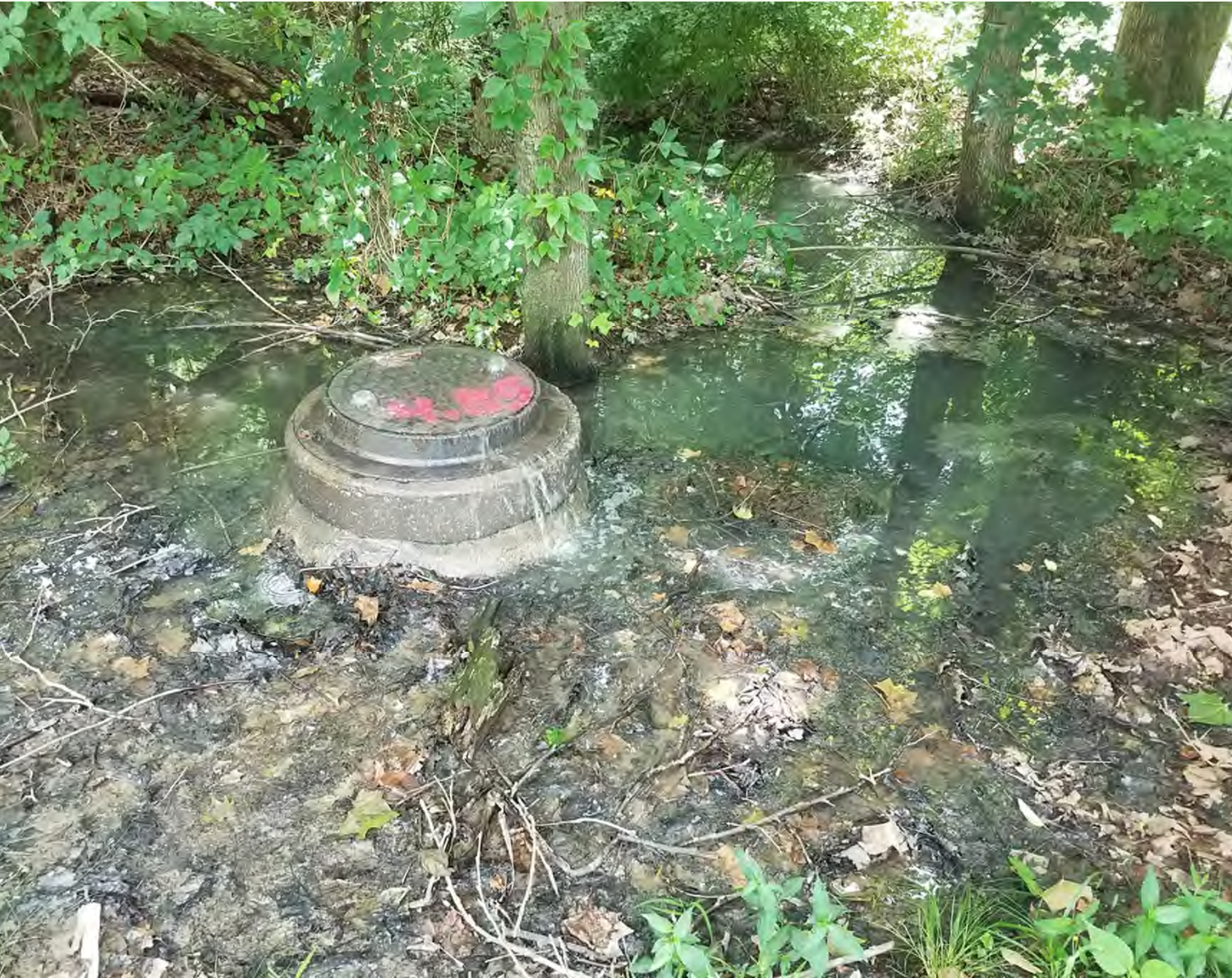
Manhole at 5730 Majestic Oak Drive
