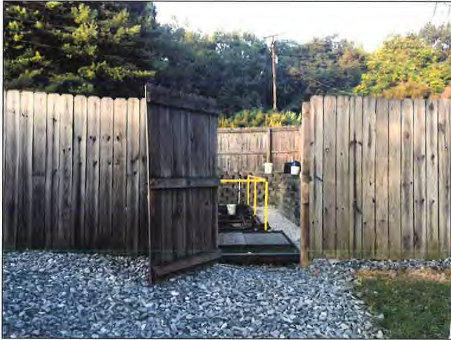
Herrington Haven WWTF
