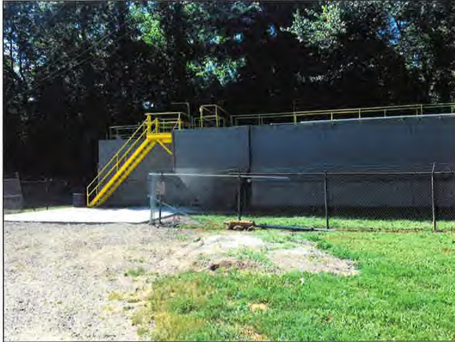
Great Oaks WWTF
