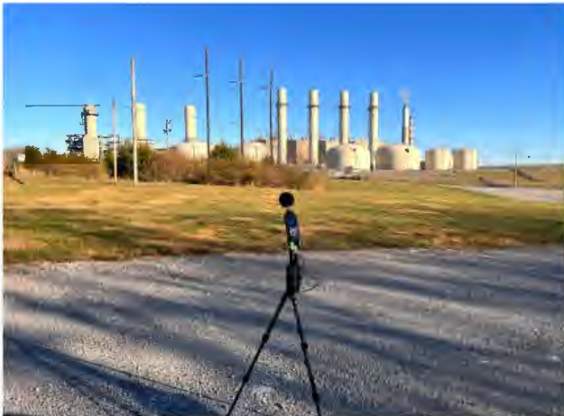
Photo Location #5: Brown Station Western Existing Property Boundary – Curdsville Road Extension
