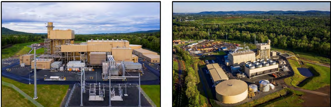
Figure 10. Proposed NGCC Unit – Reference Drone Photos (Other Facility)
