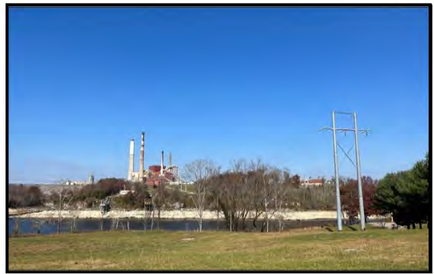
Photo Location #8: Looking northwest from the intersection of Hunter Drive/Domar Drive, across Herrington Lake.
