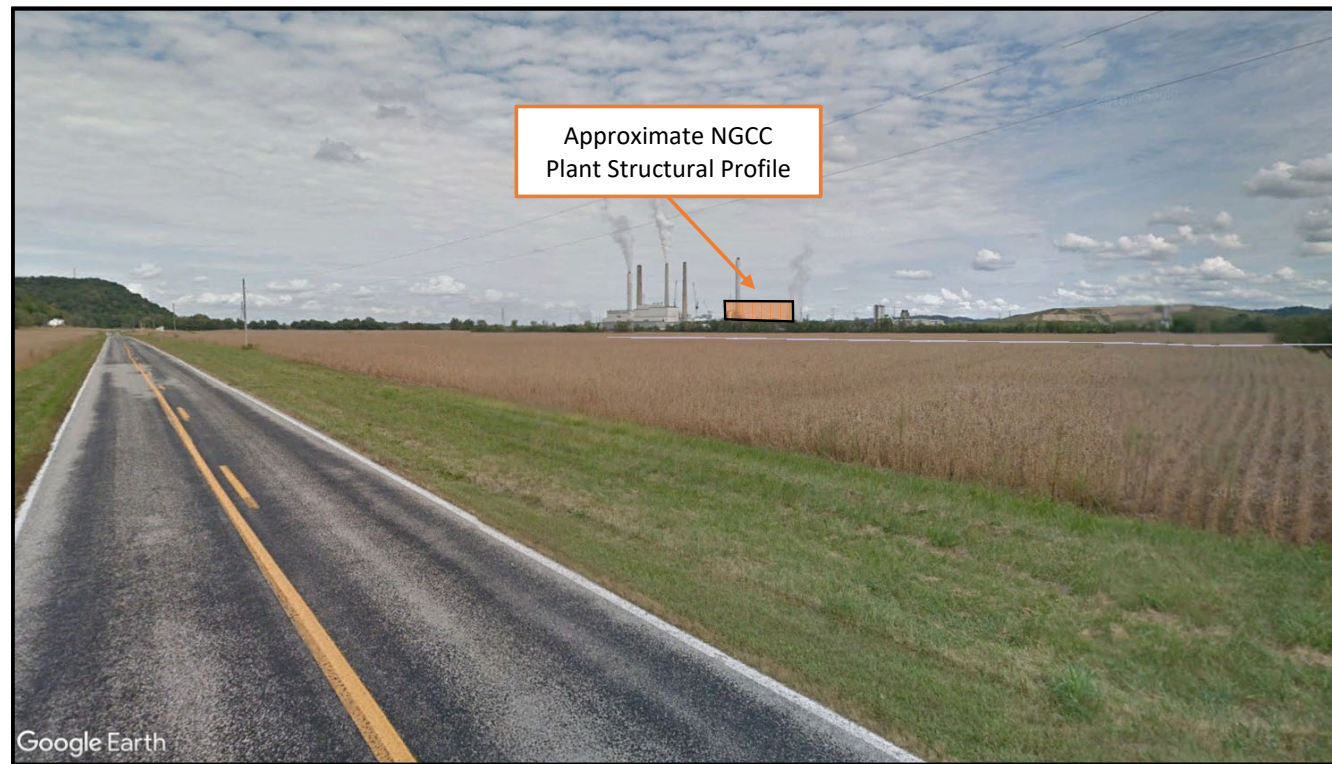
Proposed Project/NGCC Building Profile View from KY 111 (southwest of project site)
