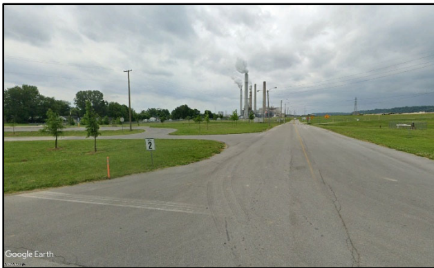
Photo Location #7: Looking south from the secondary Mill Creek Station secondary entrance along Watson Lane.
