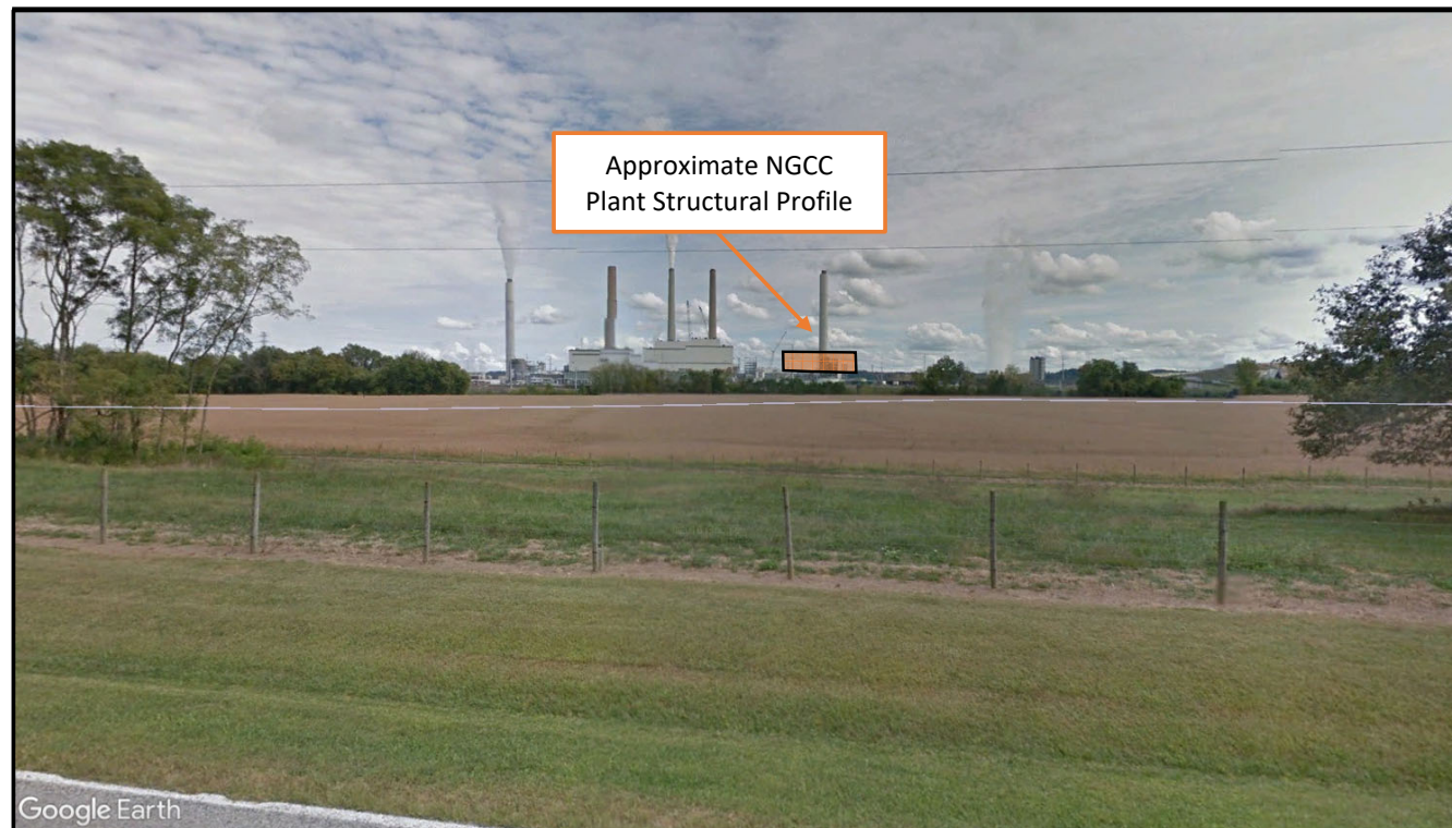
Proposed Project/NGCC Building Profile View from KY 111 (west of project site)
