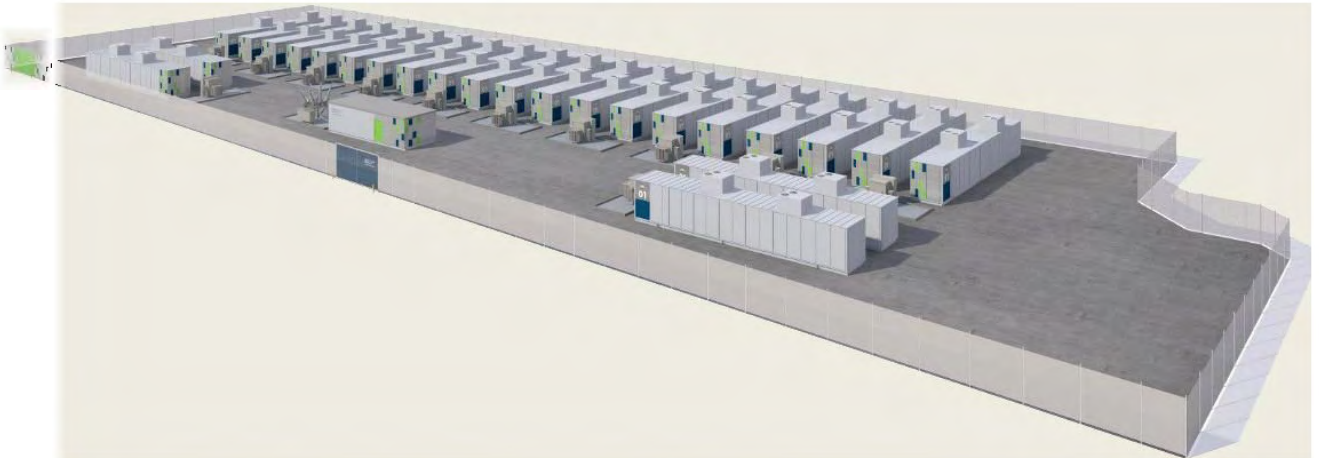
Figure 5: Typical 30 MW, 120 MWh Lithium-Ion Energy Storage Site 13
