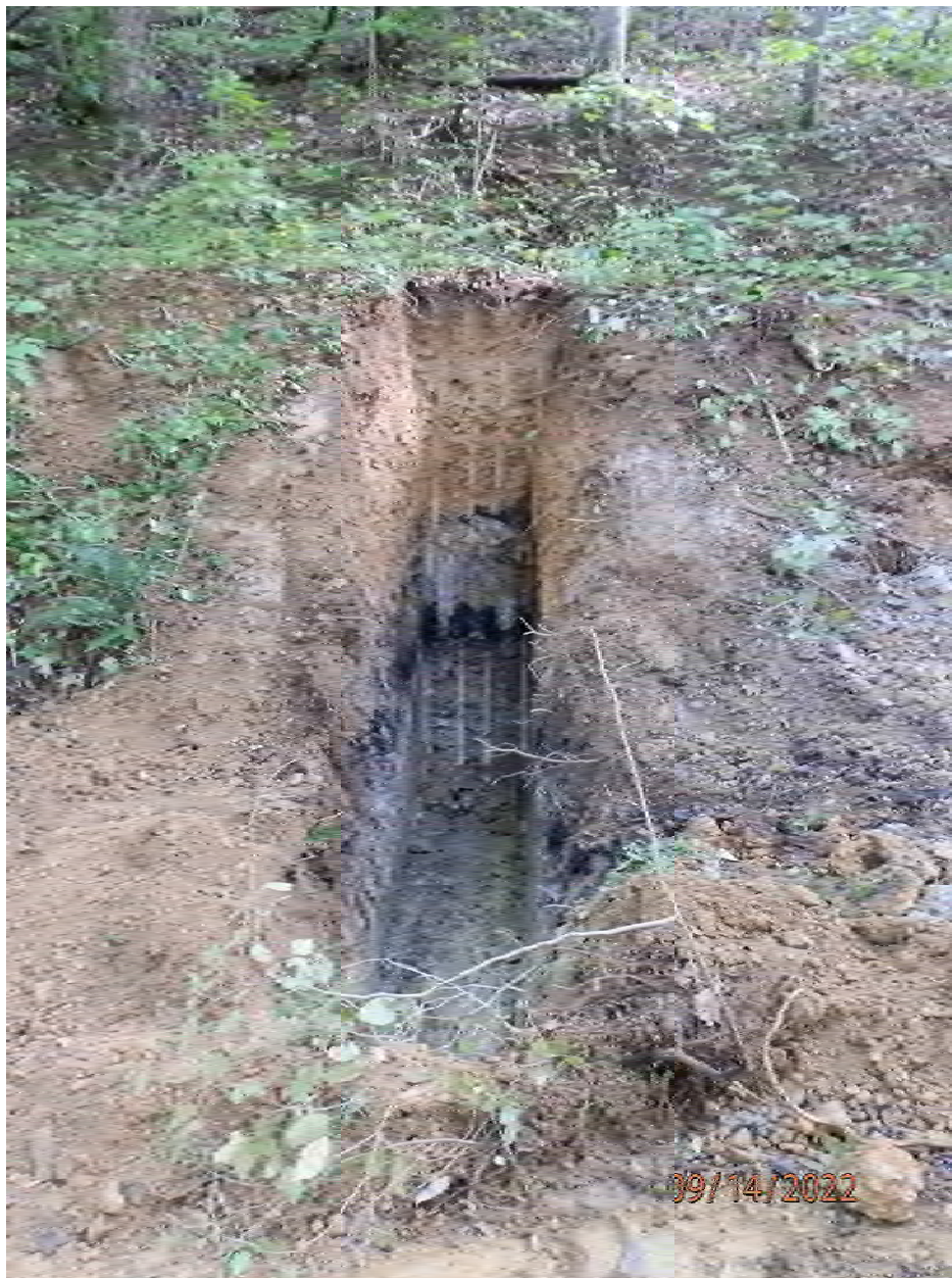
Photograph B – Standing at bottom of Trench #2, looking east uphill
