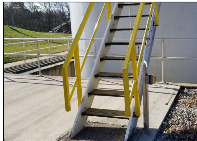
Figure #7 – Bottom of Clarifier Stairs
