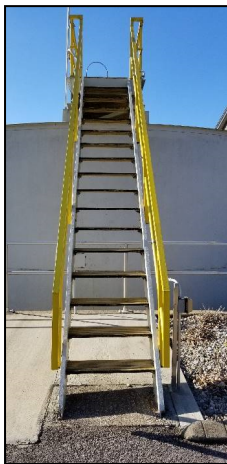
Figure #6 – Clarifier Stairs
