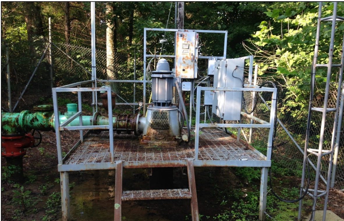
Figure #8– Gray Lane Raw Water Pump Station
