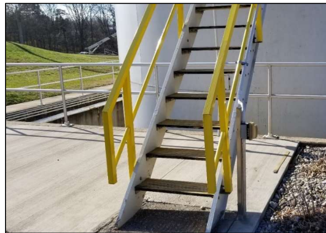
Figure #7 – Bottom of Clarifier Stairs
