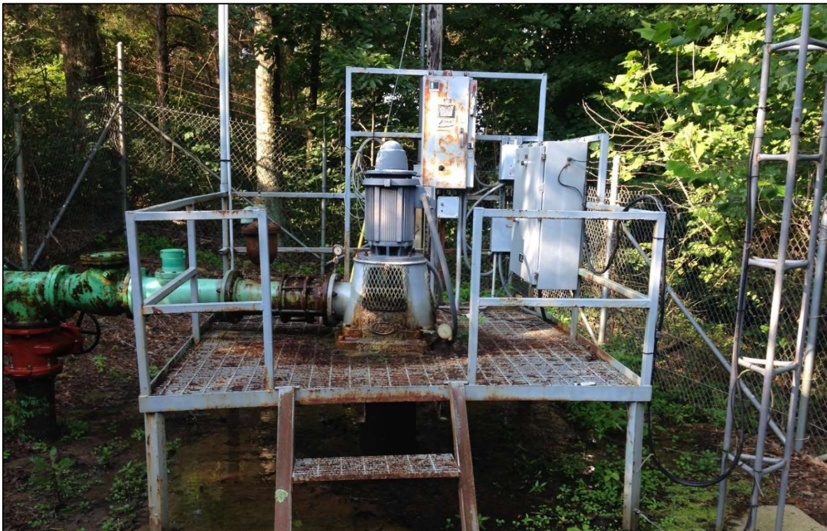
Figure #9 – Gray Lane Raw Water Pump Station
