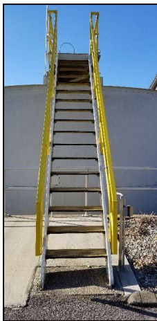
Figure #6 – Clarifier Stairs
