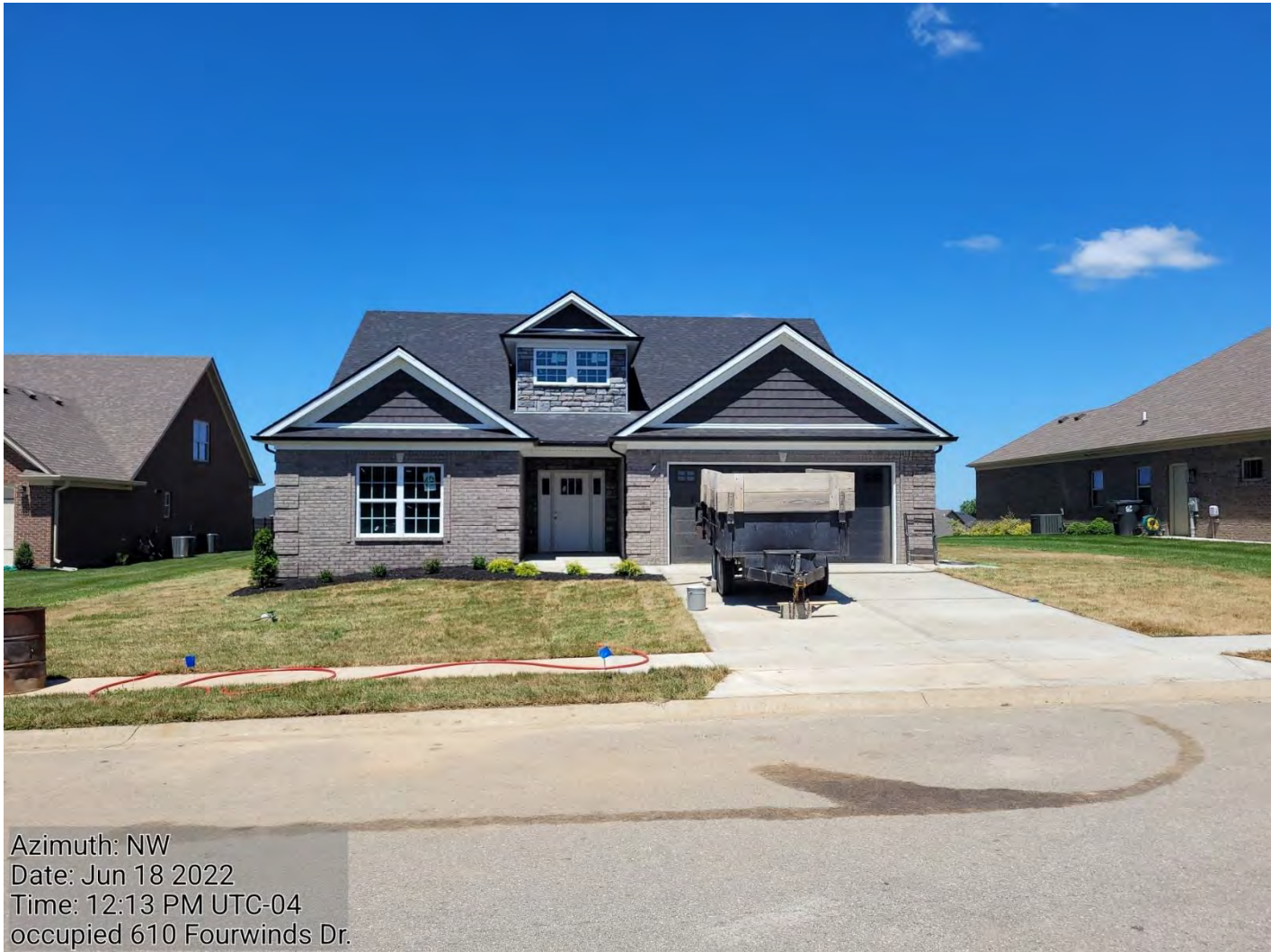
Figure 24: Building within the AOI (NV5 Field Photo)
