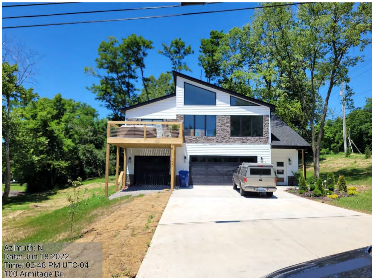
Figure 38: New modern residential structure within the AOI (NV5 Field Survey)
