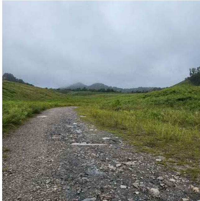
Exhibit 2.3 – Unpaved Internal Roadway
