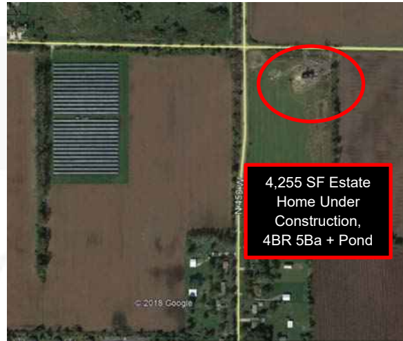
Portage Solar Farm, IN October 2016
