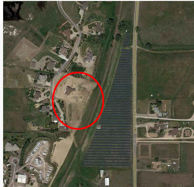
Brighton PV Solar, Adams County, CO June 2017
