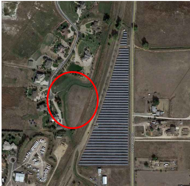
Brighton PV Solar, Adams County, CO June 2016
