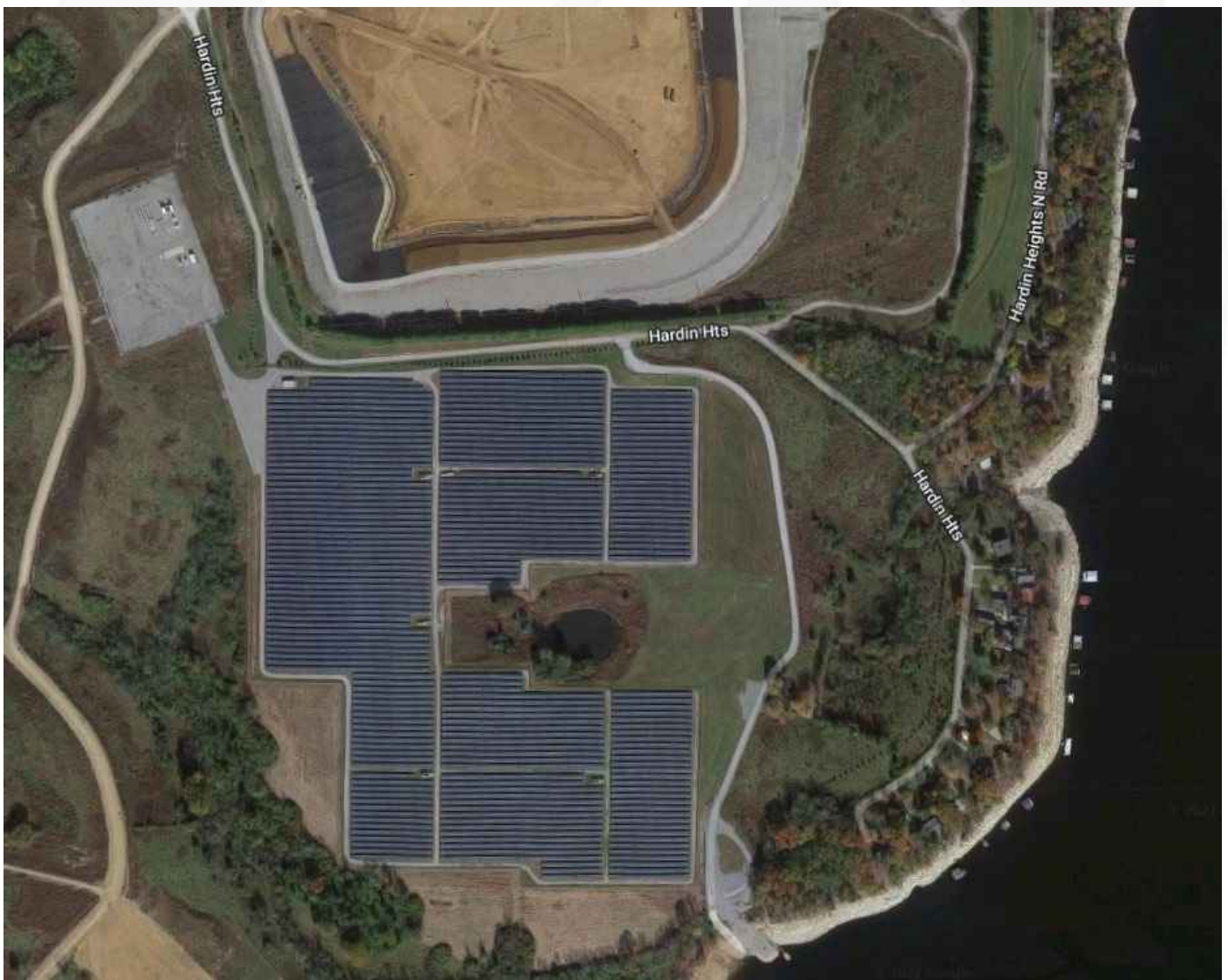
E.W. Brown Generating Station Solar Field
