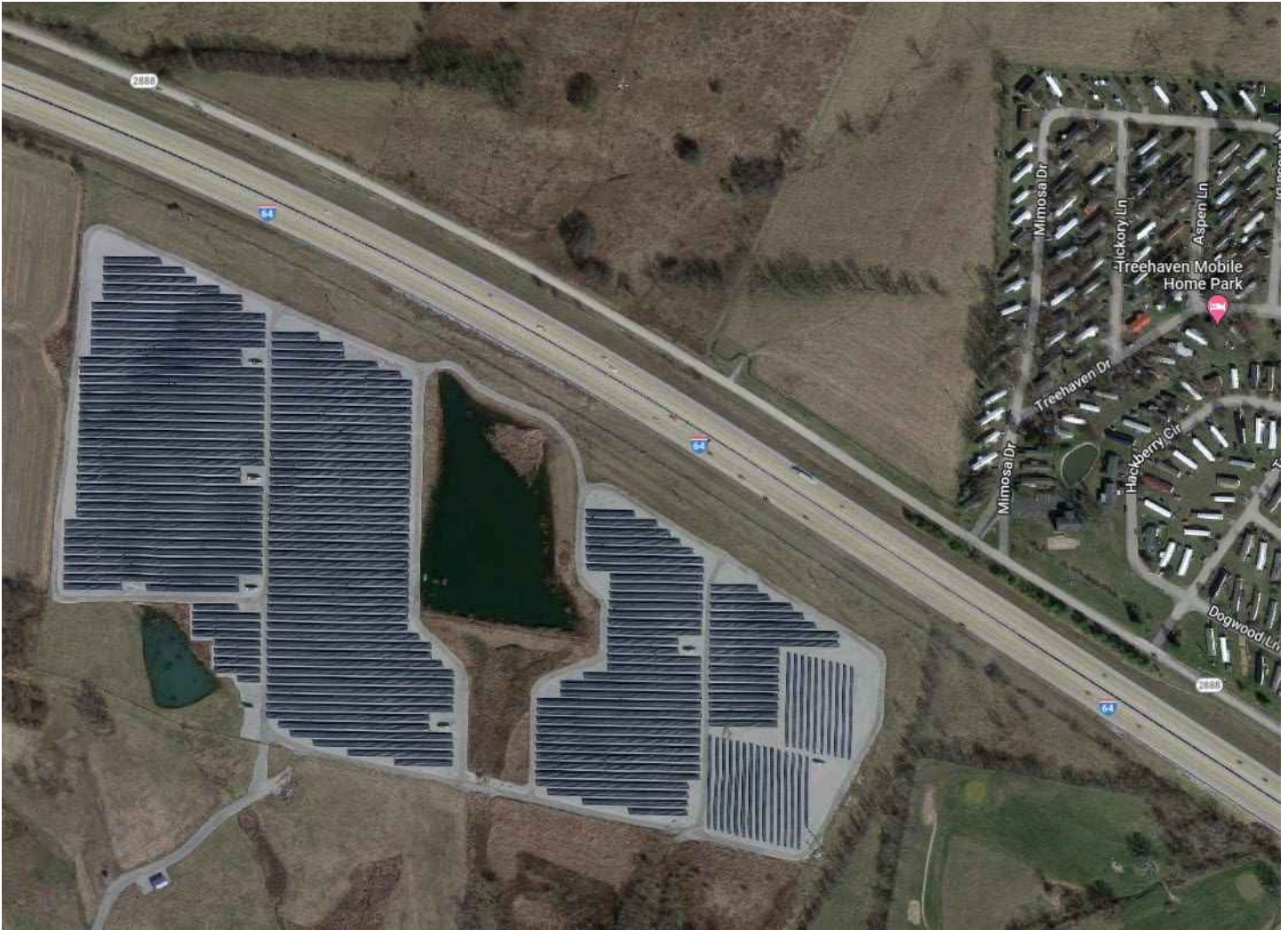
East KY Power Coop Solar Field
