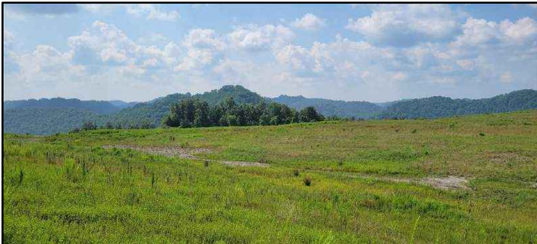
Photo 6: Overview of completed land reclamation within the subject property.
