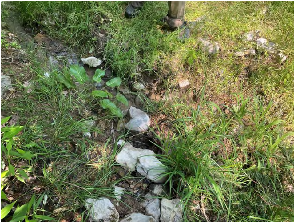
Photo 60. Stream 66-ST003 – Downstream
