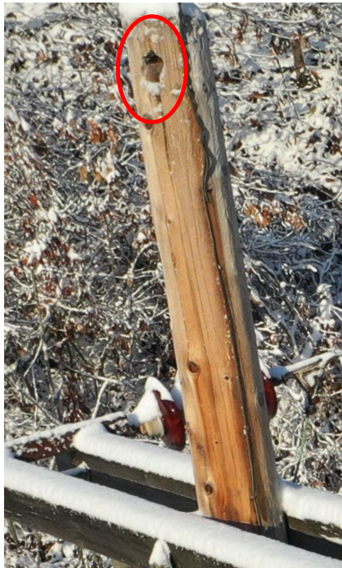
Structure K426-11: - Pole Cavity
