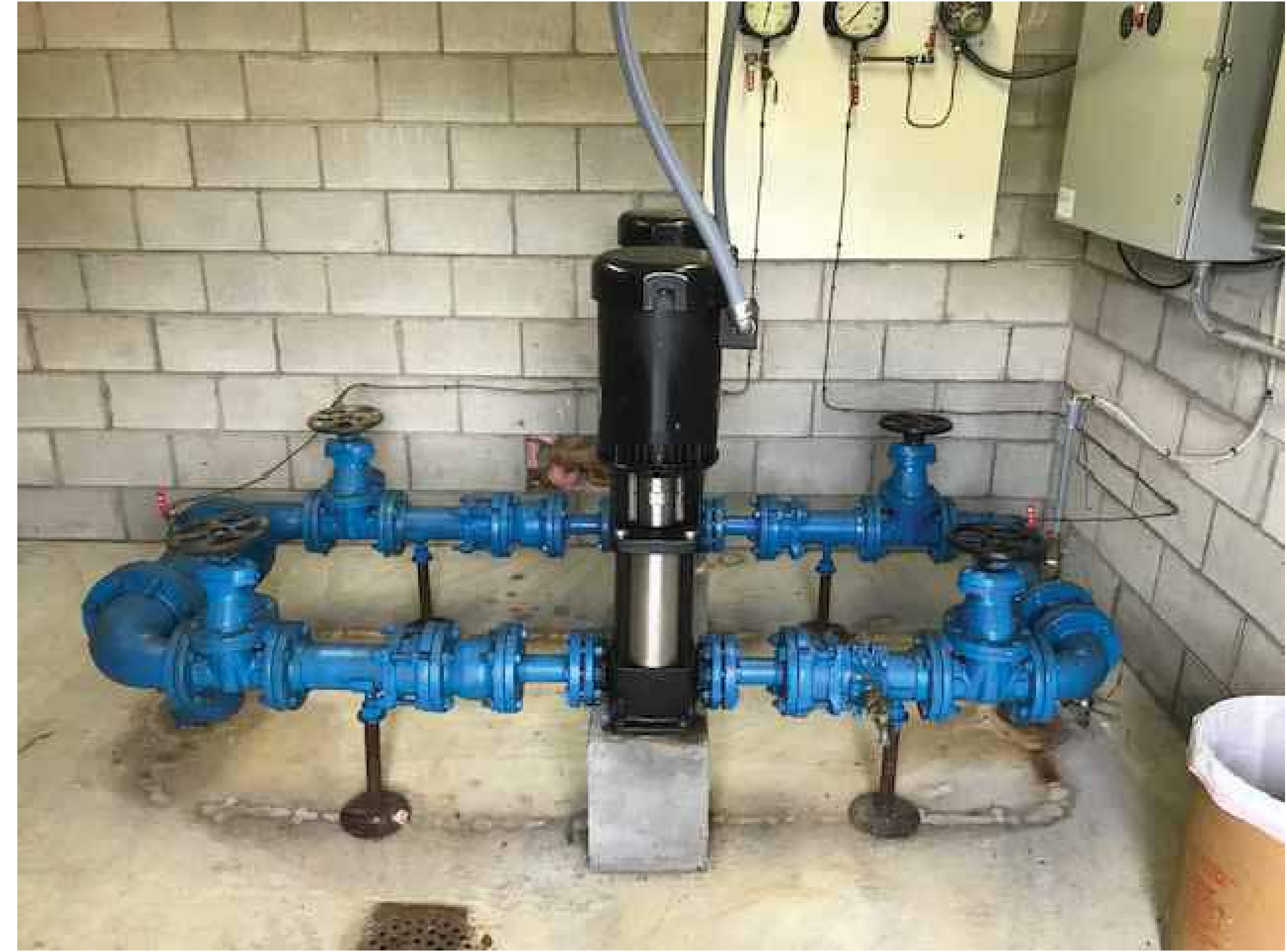
ELEVATION VIEW - EX. KY 7 BOOSTER PUMP STATION
