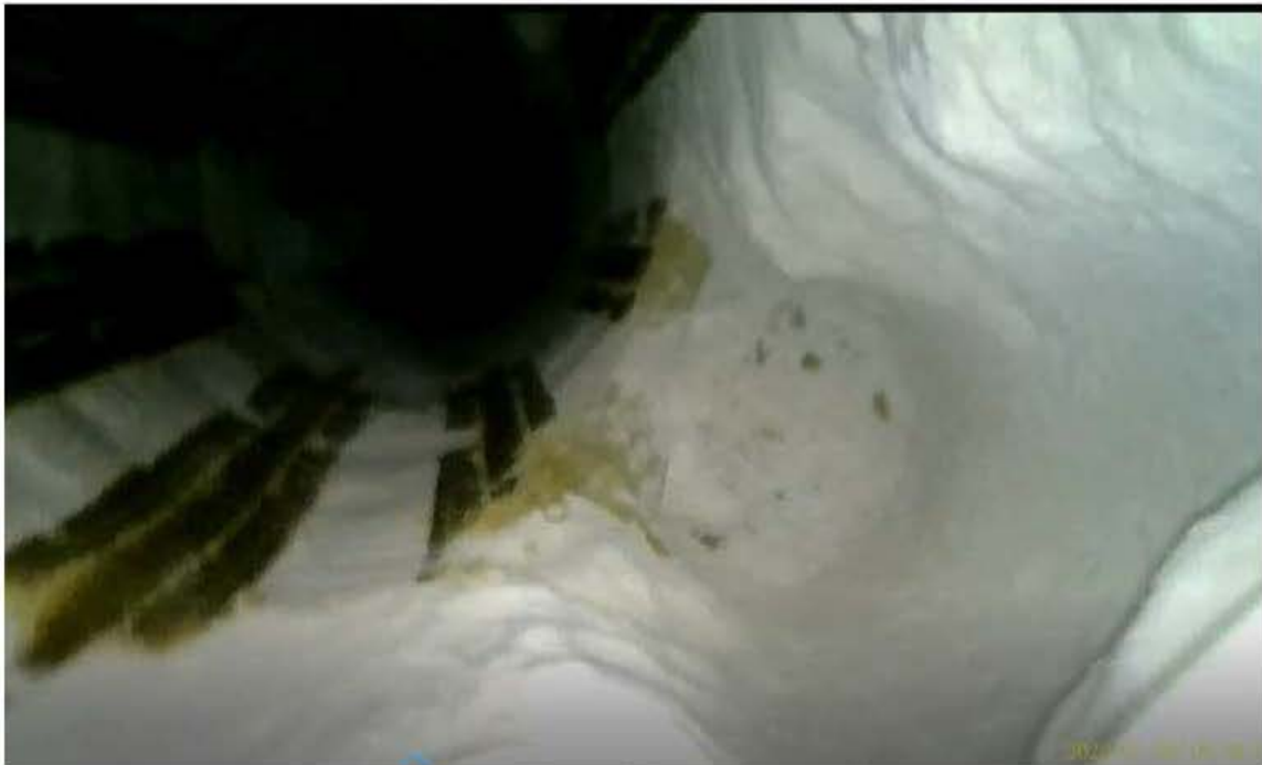
Void Near Siltstone/Limestone Interface
