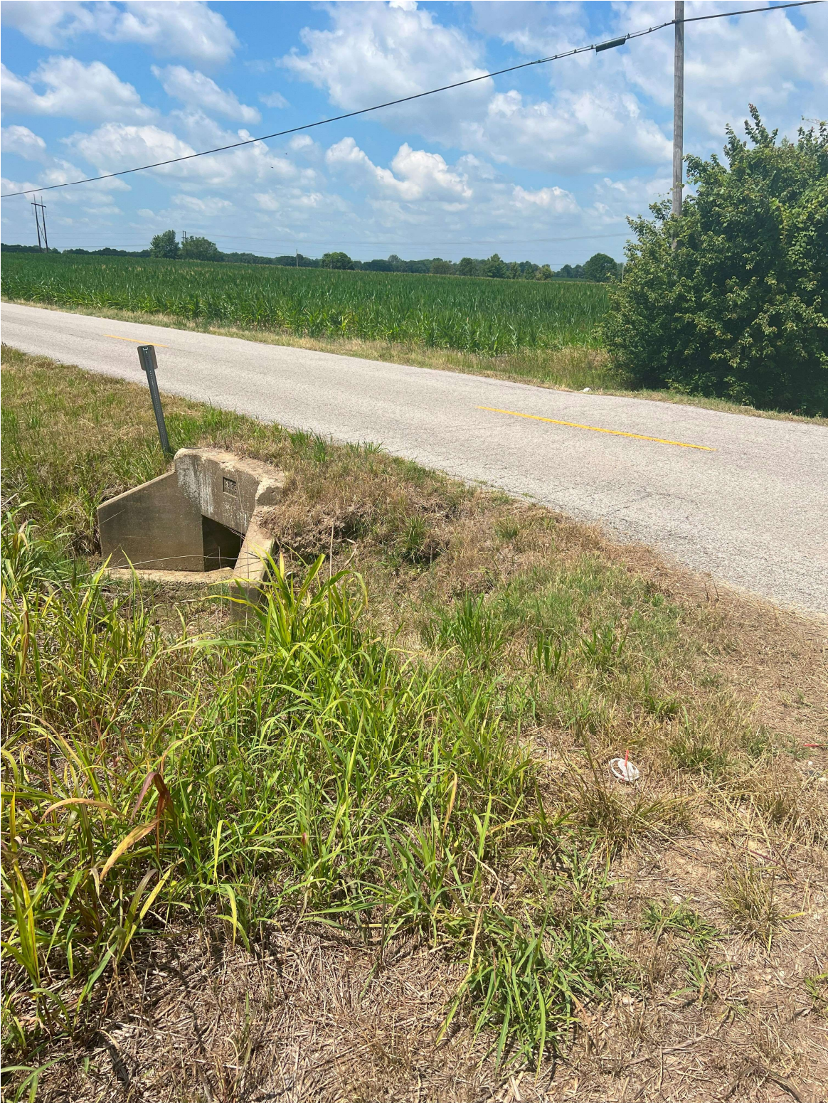
Picture (9) Location #1 (Culvert under KY-283)
