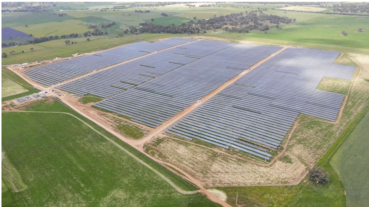
Picture (3) Solar Modules Installed on Farmland 3
