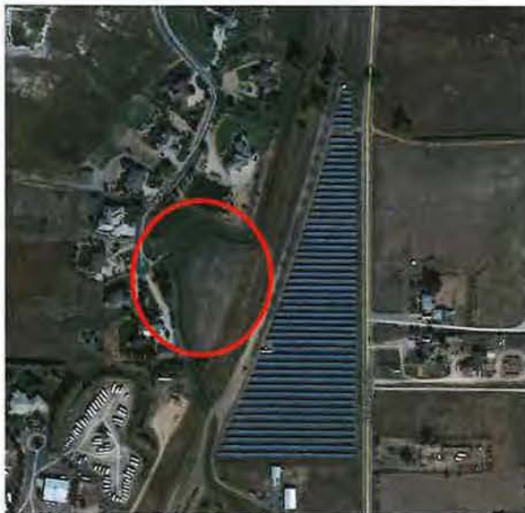
Brighton PV Solar, Adams County, CO June 2016
