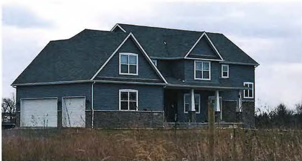
4,255 square foot estate home under construction, adjacent to Portage Solar Farm located in Indiana On-site pond and attached garage (cost estimated at $465,000) April 2018
