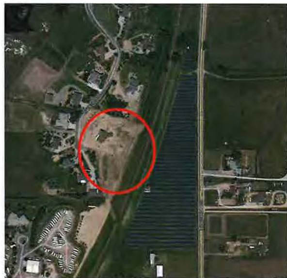
Brighton PV Solar, Adams County, CO June 2017
