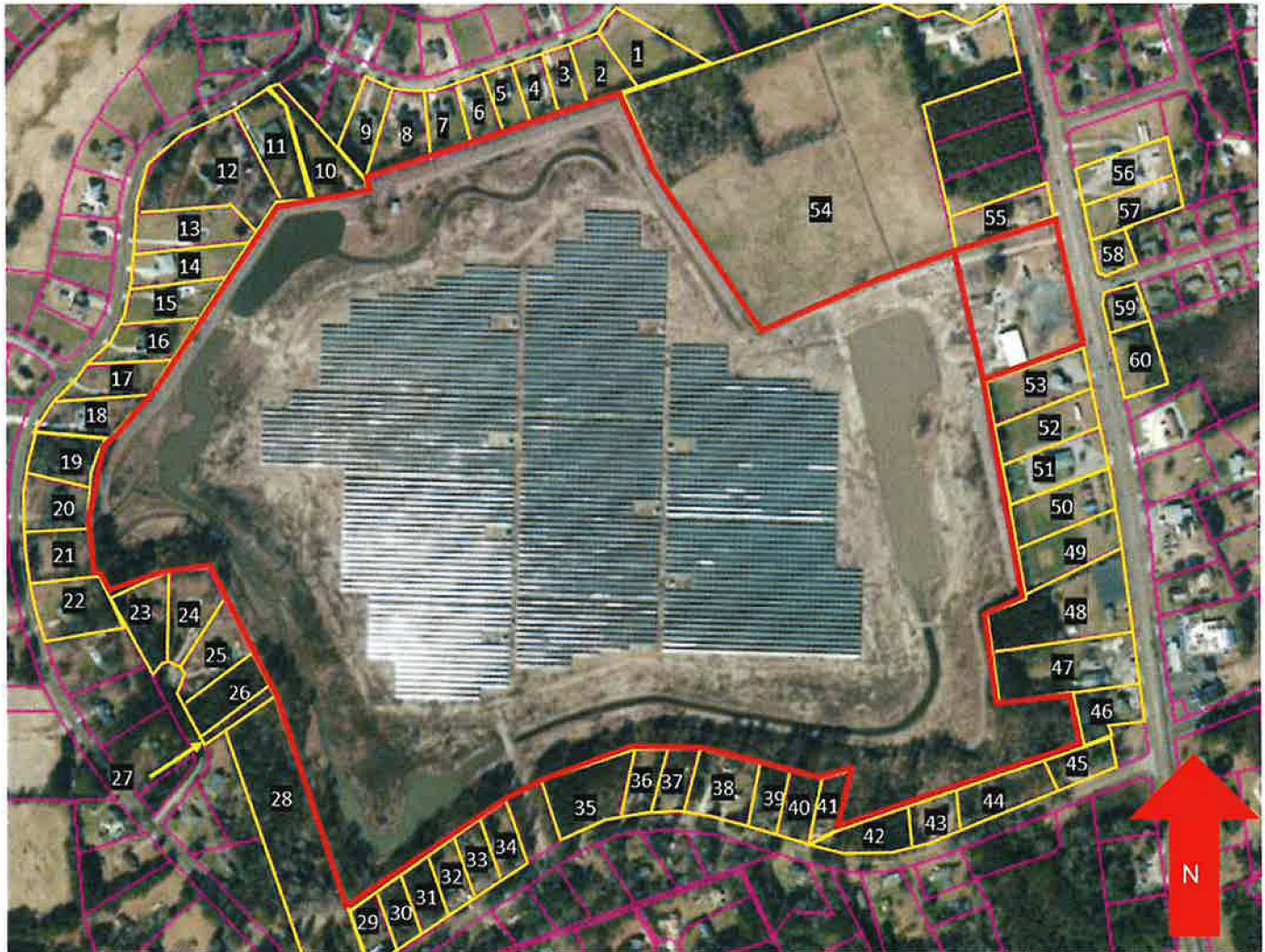
Sunshine Farms Solar – Adjoining Properties
