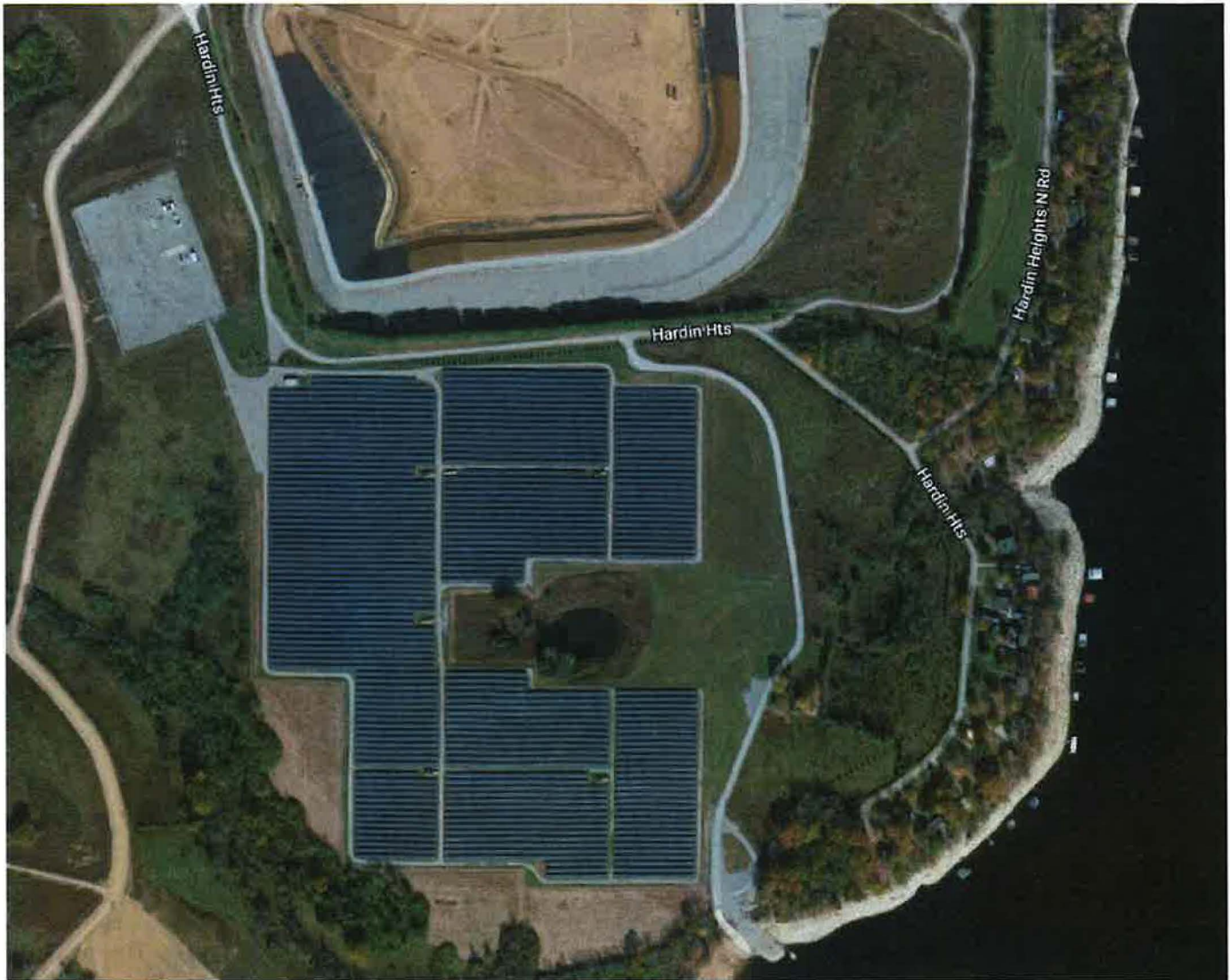
E.W. Brown Generating Station Solar Field
