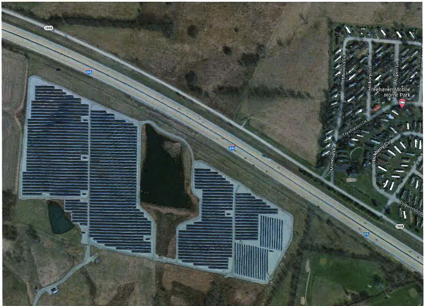
East KY Power Coop Solar Field
