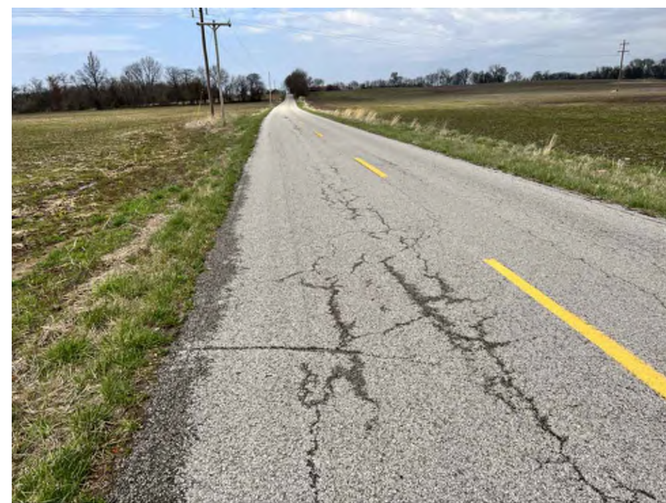
SITE ENTRANCE # 208 Northwestbound KY1299
