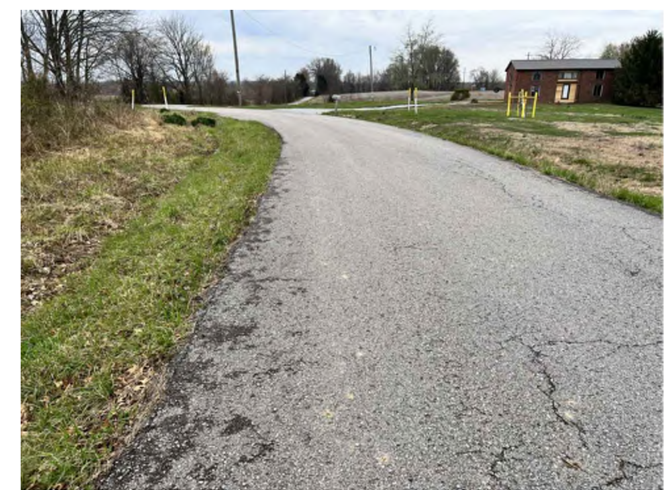
SITE ENTRANCE # 202 Southbound W N Royster Road
