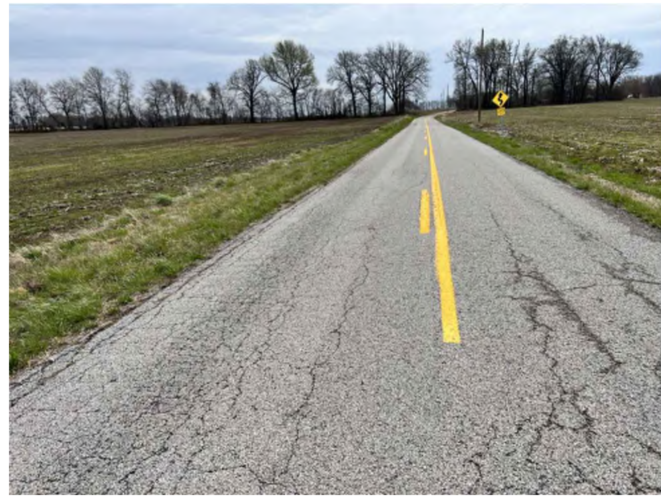
SITE ENTRANCE # 208 Southeastbound KY1299
