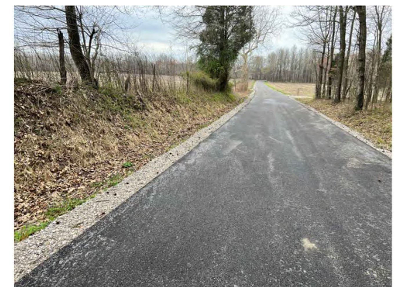
SITE ENTRANCE # 207 Southbound Thomason Rd
