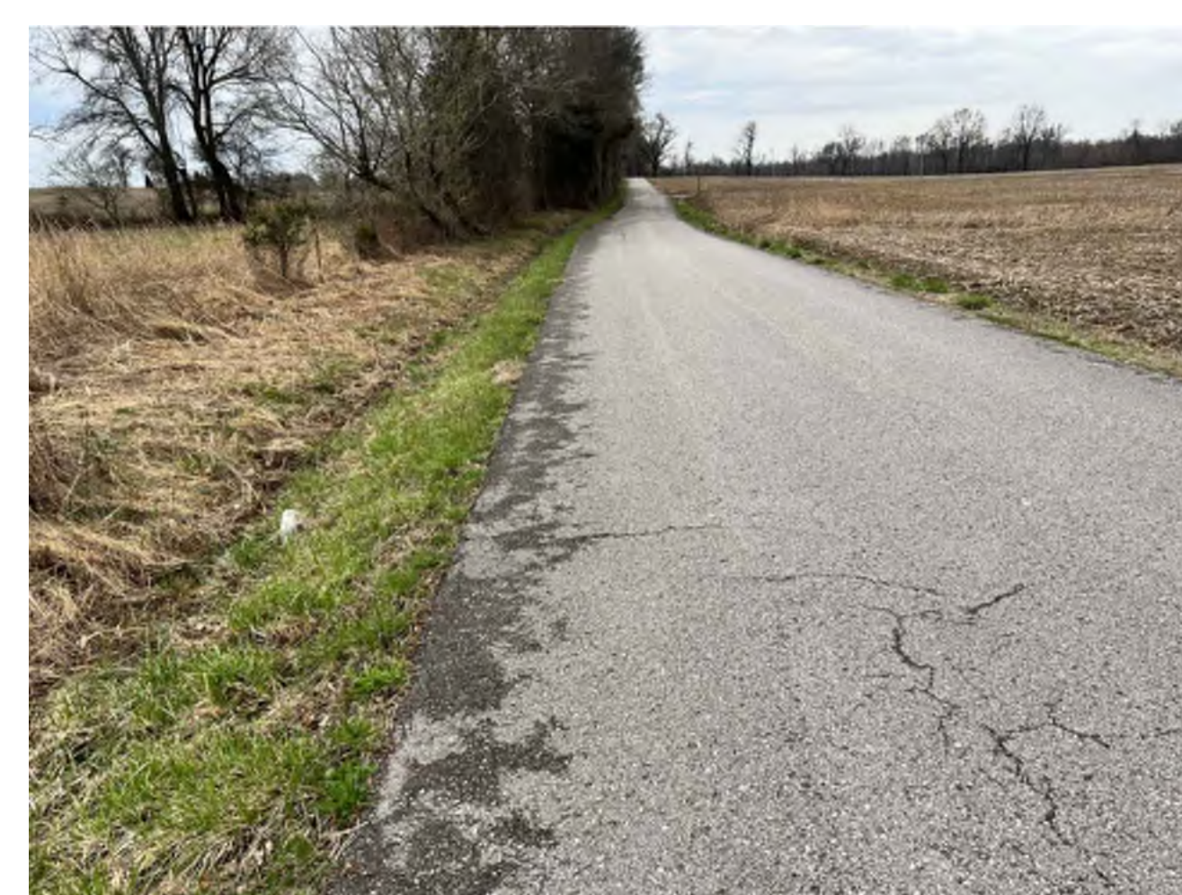
SITE ENTRANCE # 201 Southbound W N Royster Road
