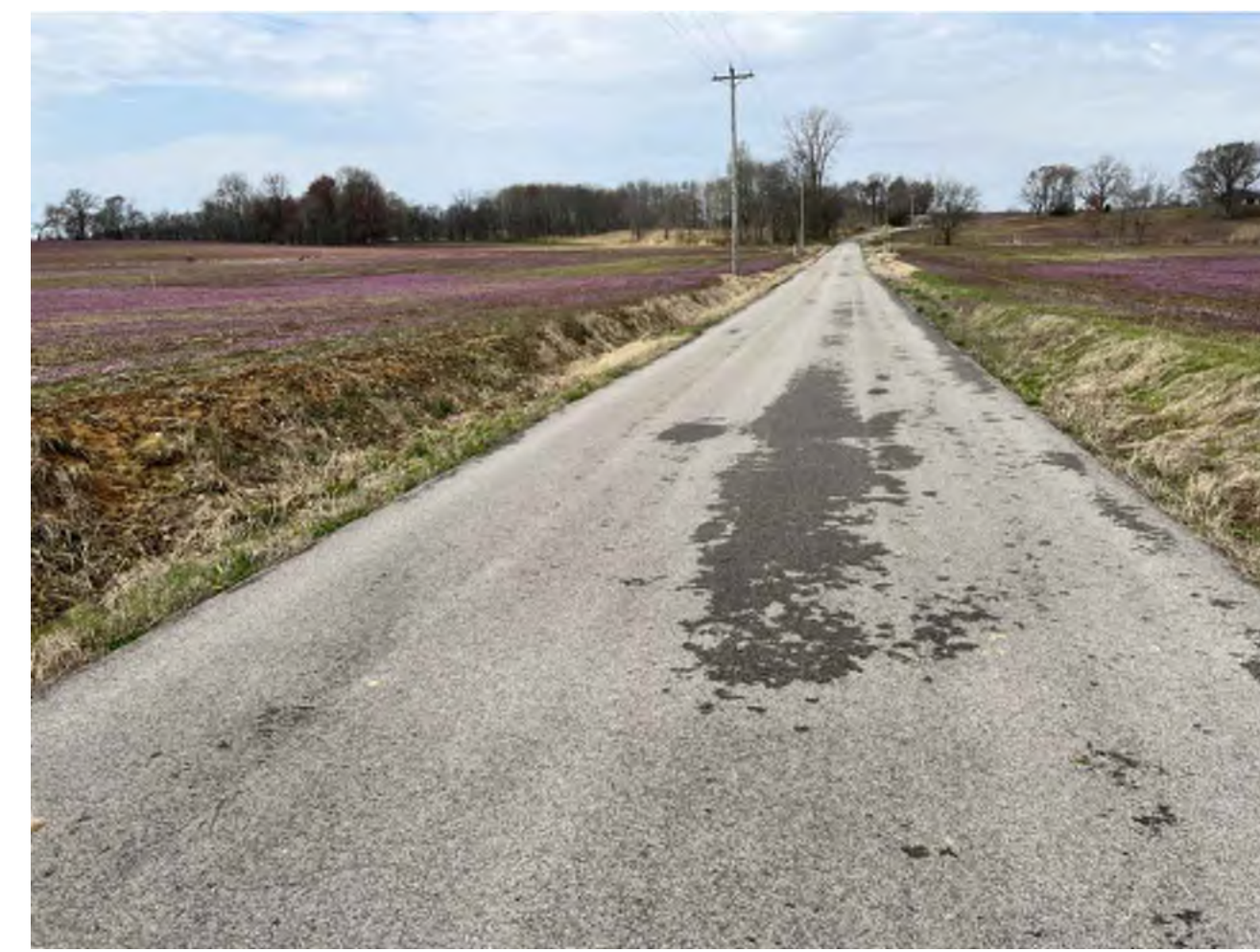
SITE ENTRANCE # 212 Westbound Cherry Hill Rd
