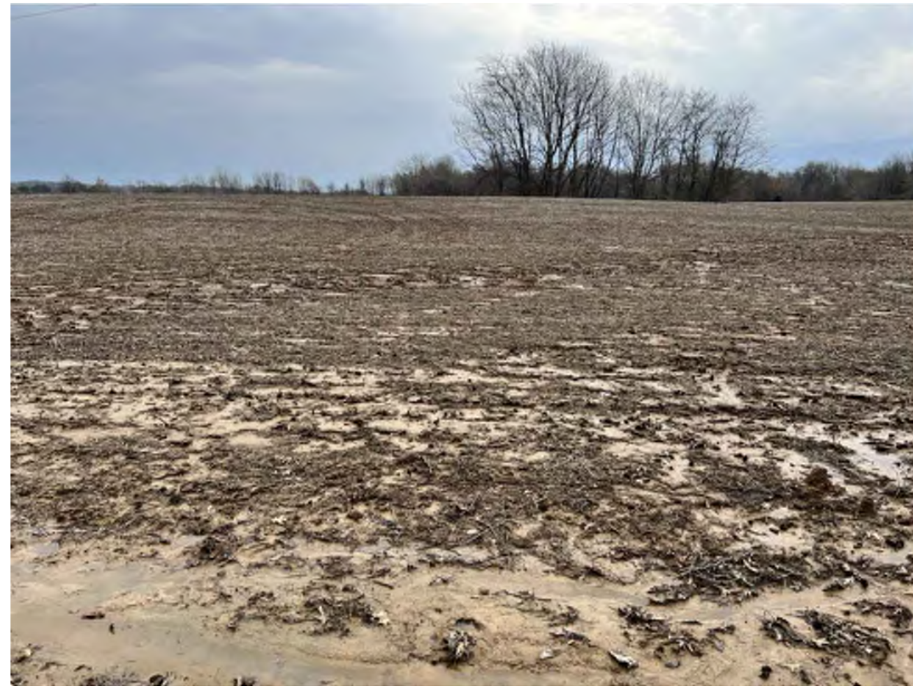
SITE ENTRANCE # 205 A&B Eastbound Thomason Rd
