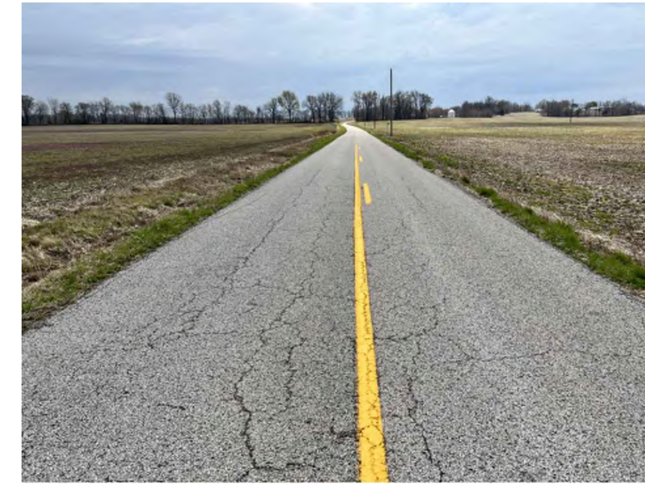
SITE ENTRANCE # 209 Southeastbound KY1299
