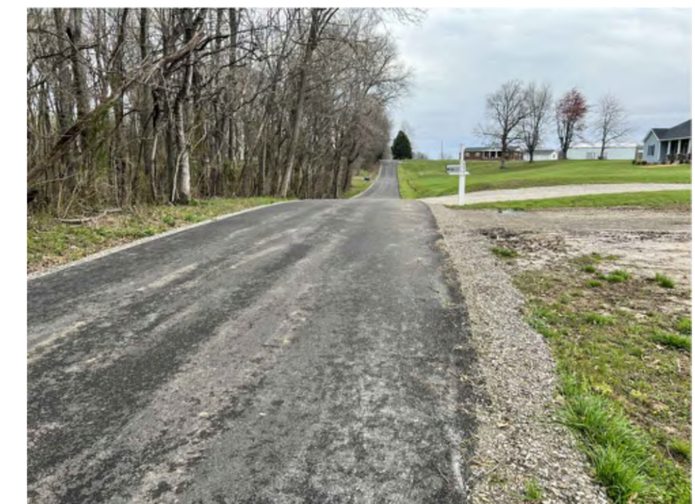
SITE ENTRANCE # 206 Northbound Thomason Rd
