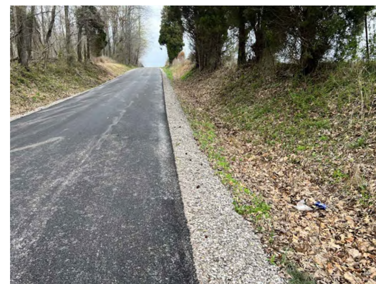
SITE ENTRANCE # 207 Northbound Thomason Rd
