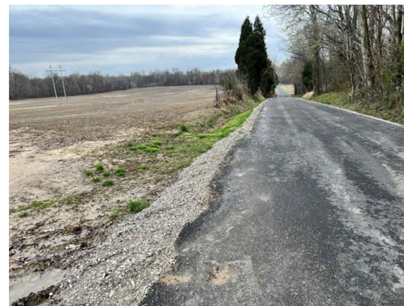
SITE ENTRANCE # 206 Southbound Thomason Rd
