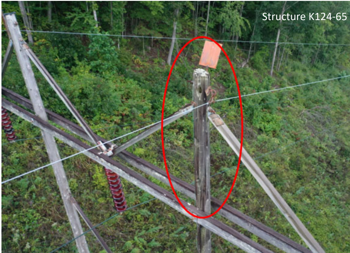
Structure K124-65: - Pole Cavity
