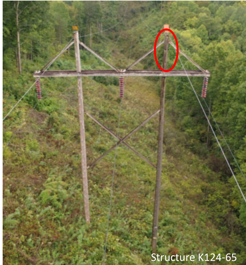
Structure K124-65: - Pole Cavity
