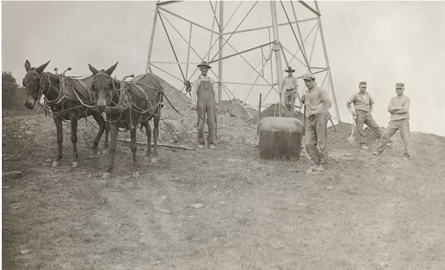
Backfilling crew on tower construction, 1925
