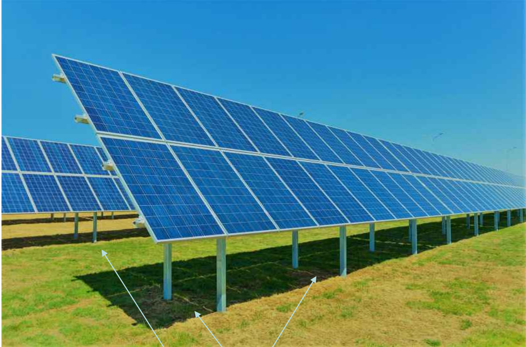
Final install of piles
