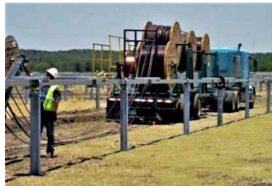
Installing Collection System
