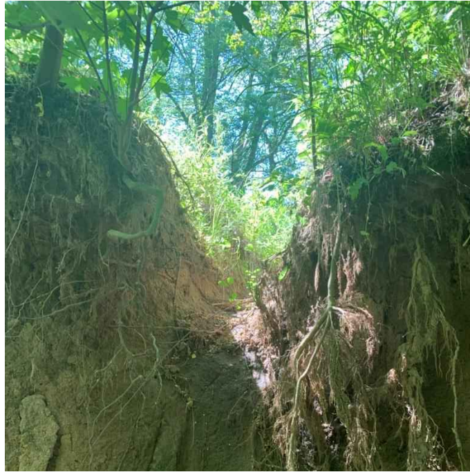
Photo 7: Karst feature 1 located along a fencerow within the central portion of the Project area.
