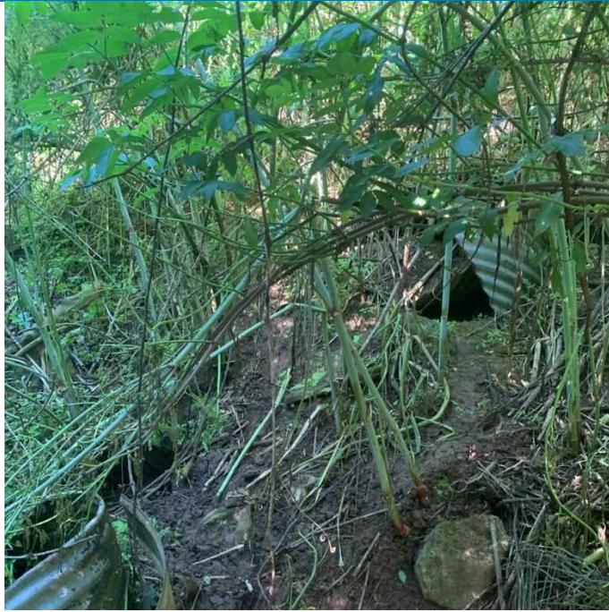
Photo 9: Karst feature 2 located within a hayfield within the southern portion of the Project Area.
