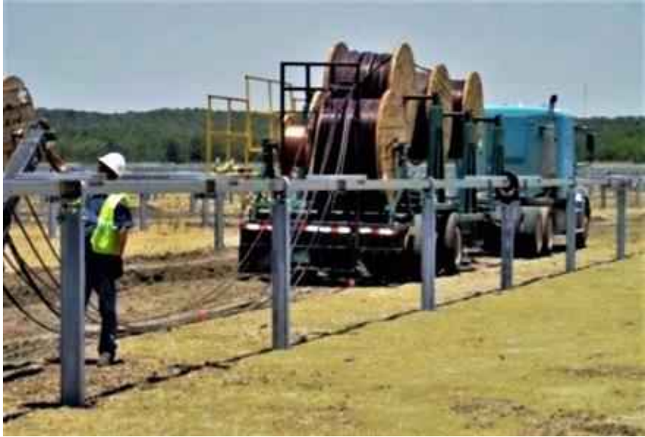
Typical Collection Line Installation
