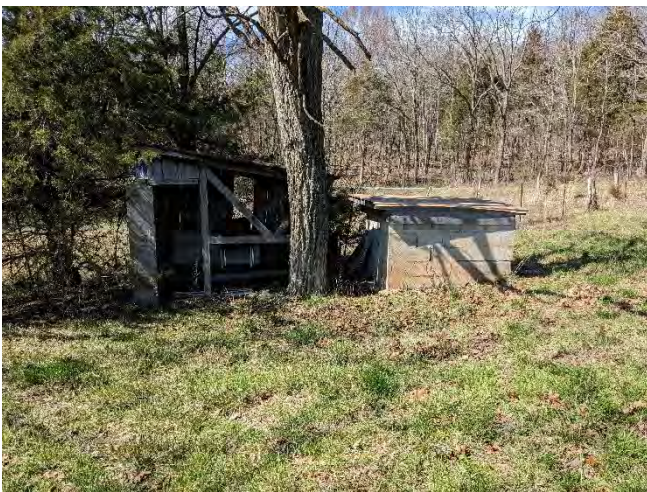
Photo 11: Various outbuildings near structures off of Rowletts Cave Road
