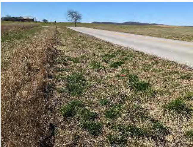
Photo 17: Typical ditches within throughout the subject property
