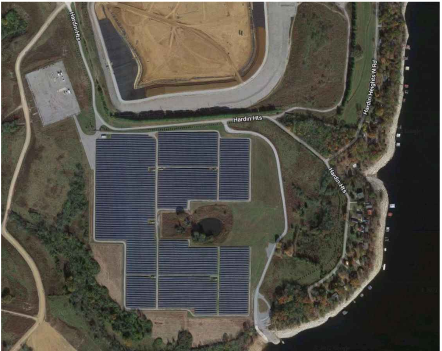
E.W. Brown Generating Station Solar Field
