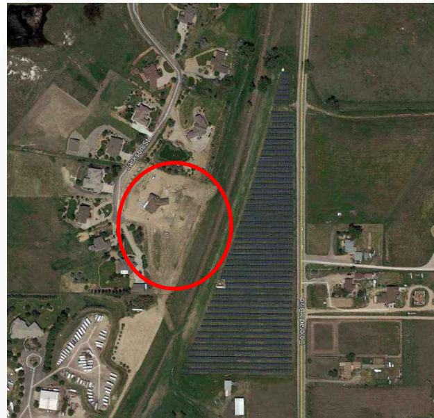
Brighton PV Solar, Adams County, CO June 2017
