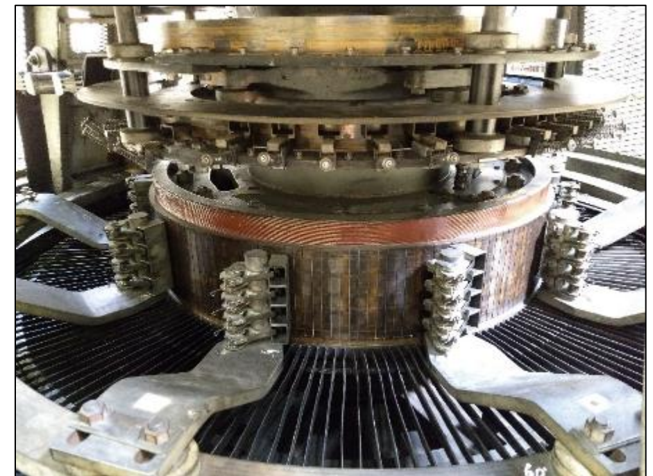
Rotating Exciter at Old Hickory
