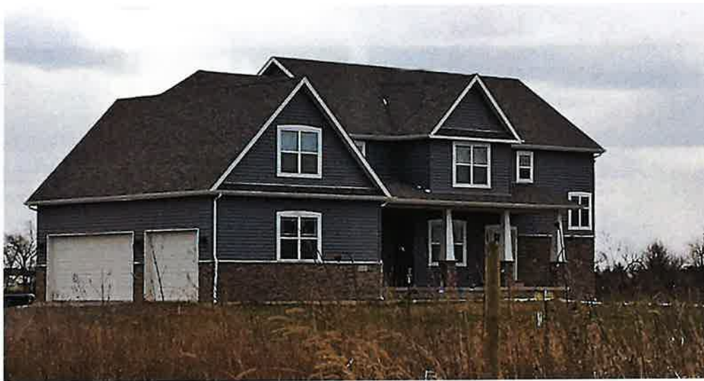
4,255 square foot estate home under construction, adjacent to Portage Solar Farm located in Indiana
