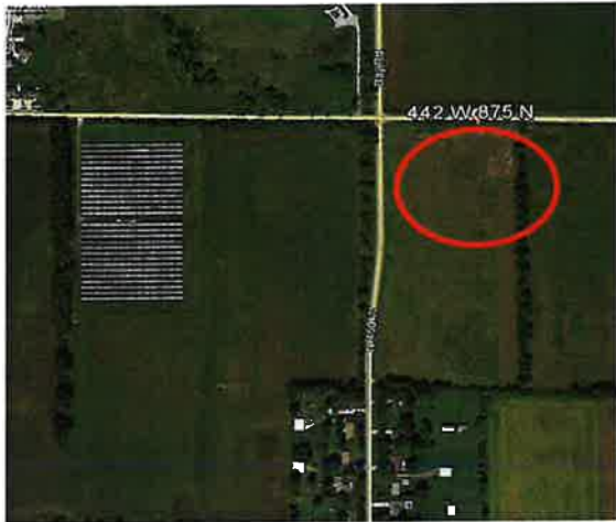
Portage Solar Farm, IN October 2015
