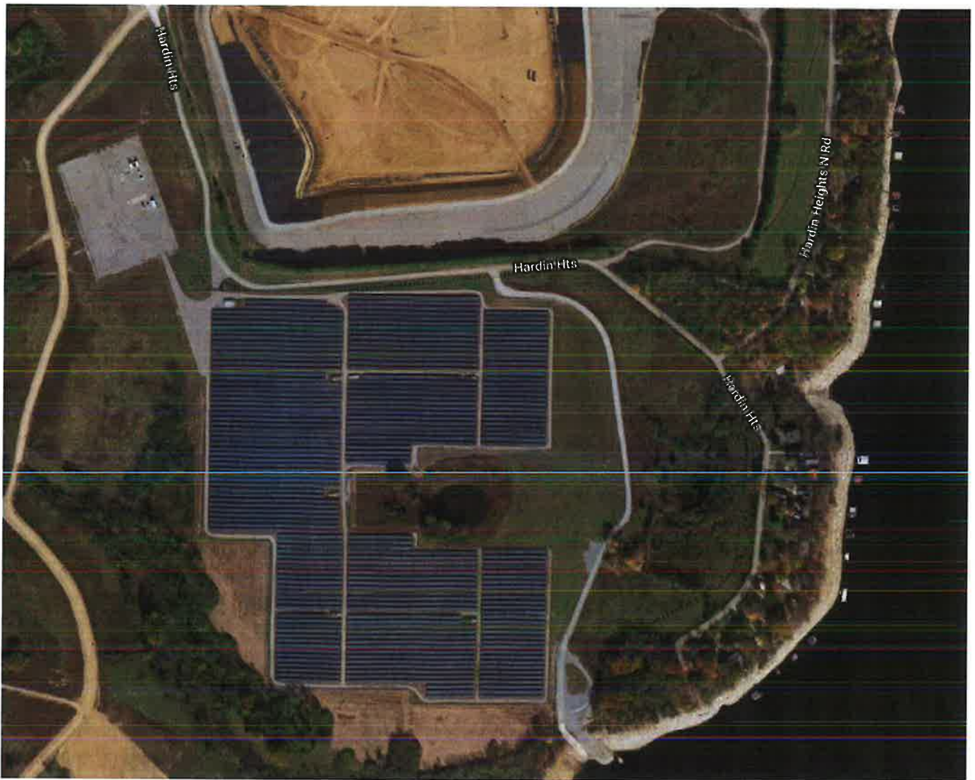
E.W. Brown Generating Station Solar Field
