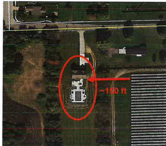
Dominion Indy III Solar Farm October 2016
