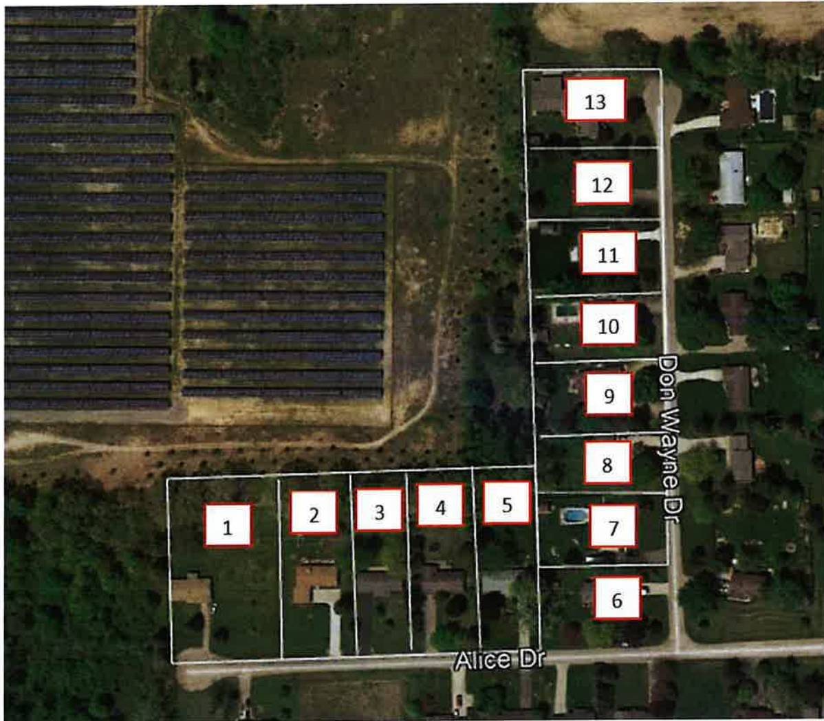
DTE's Lapeer Solar Projects - Demille Adjoining Properties
