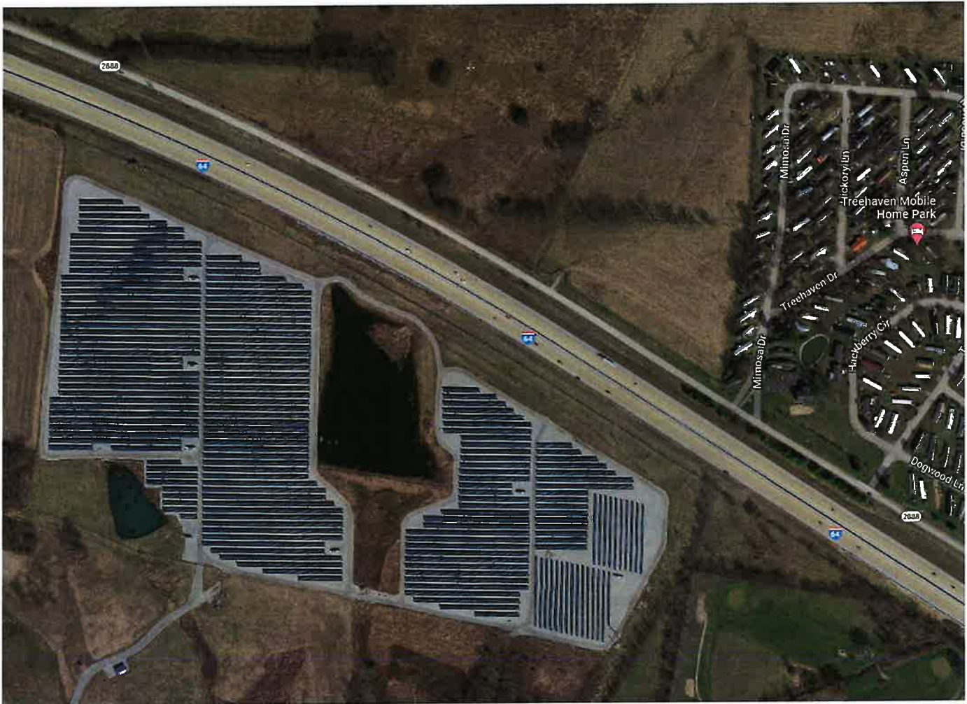
East KY Power Coop Solar Field
