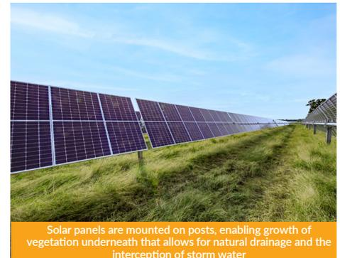
Solar panels are mounted on posts, enabling growth of vegetation underneath that allows for natural drainage and the interception of storm water
